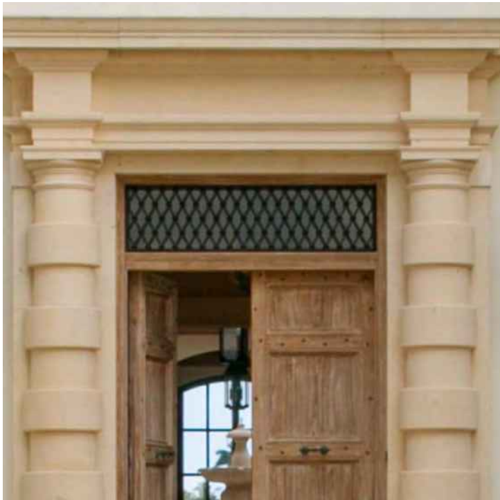
STONE SURROUNDS & DETAILS; LIMED WOOD & METAL GRILLE FRONT DOOR
