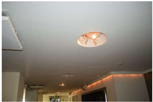
Fig. 206. Detail of ceiling finish and recessed light fixture at lobby, July 2021.
