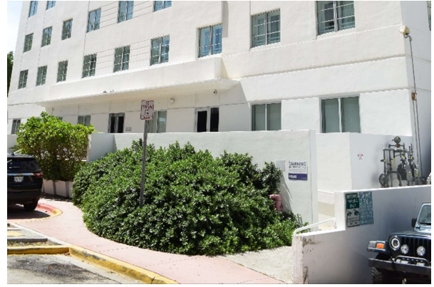
Fig. 130. Detail of planting beds and large planting pots adjacent pedestrian sidewalk in front of Cromwell, July 2021.
