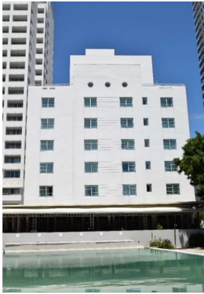
Fig. 195. View of east elevation, July 2021.
