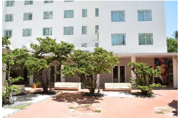
Fig. 200. Detail of first level of south elevation, July 2021.
