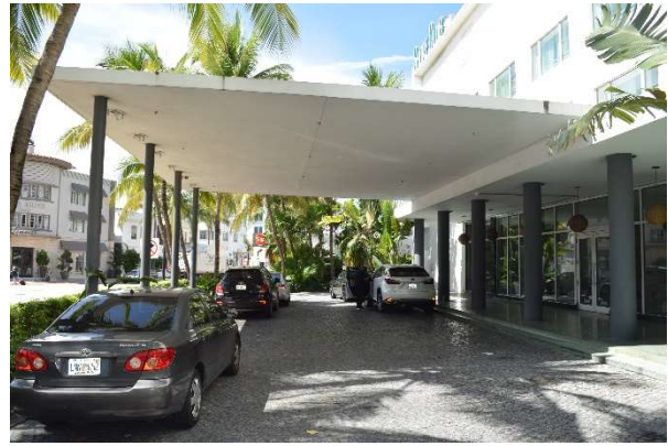
Fig. 153. Detail of porte-cochere at west elevation, July 2021.
