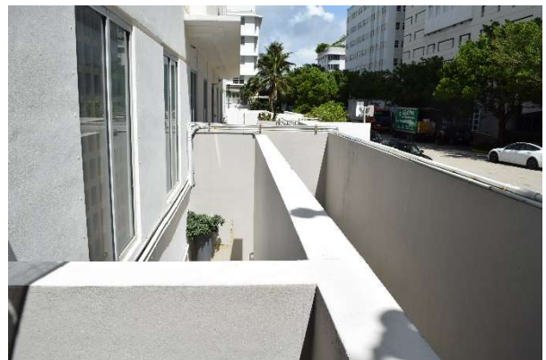
Fig. 128. Detail of areaway to basement level at east end of north elevation of Cromwell, July 2021.
