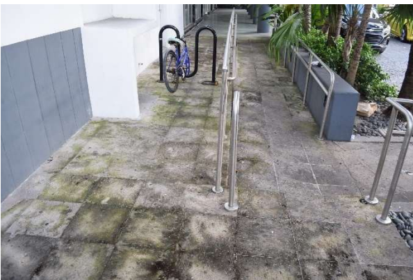
Fig. 123. Detail of accessible ramp and bike rack, July 2021.
