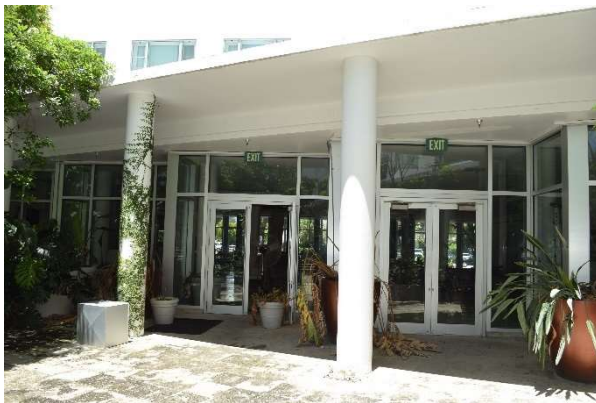
Fig. 161. Detail of storefront at courtyard area, July 2021.
