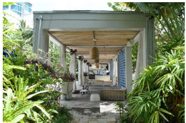
Fig. 141. Detail of pavilion adjacent main pool, July 2021.
