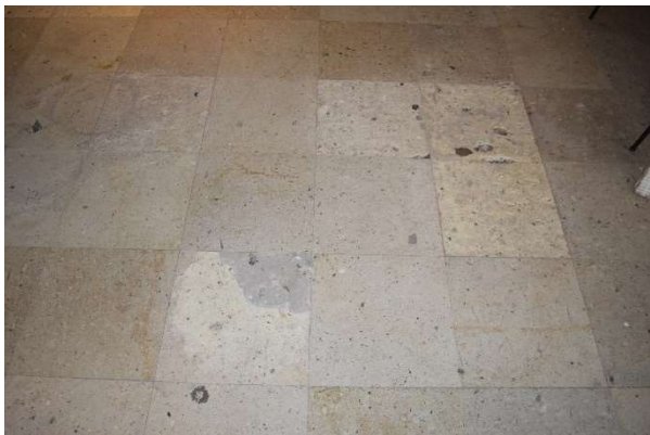
Fig. 205. Detail of flooring in lobby, July 2021.
