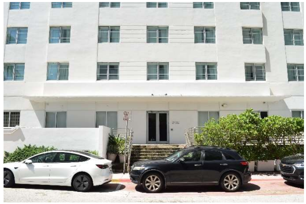
Fig. 192. Detail of base and stairs at north elevation entrance, July 2021.
