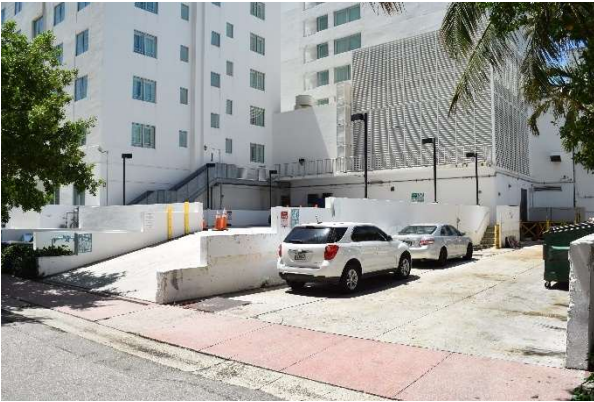
Fig. 125. View of flat drive and elevated ramp, July 2021.
