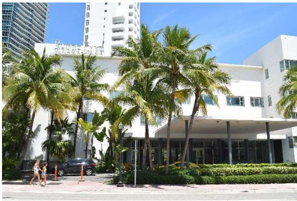
Fig. 147. View of horizontal northern block at west elevation of Shore Club, July 2021.
