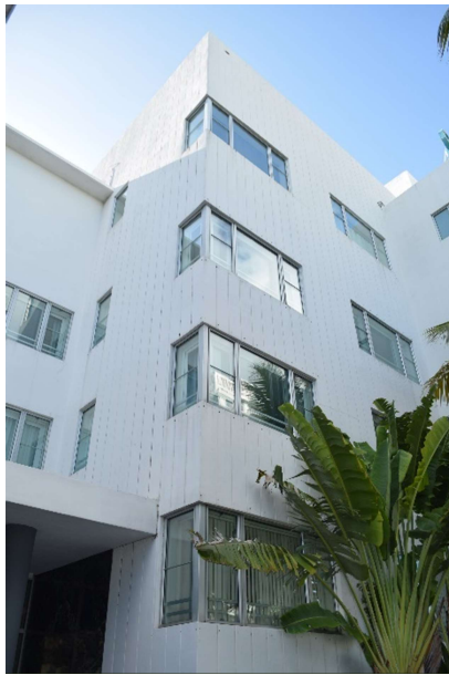
Fig. 156. Detail of vertical incised lines and corner windows at southern block, July 2021.
