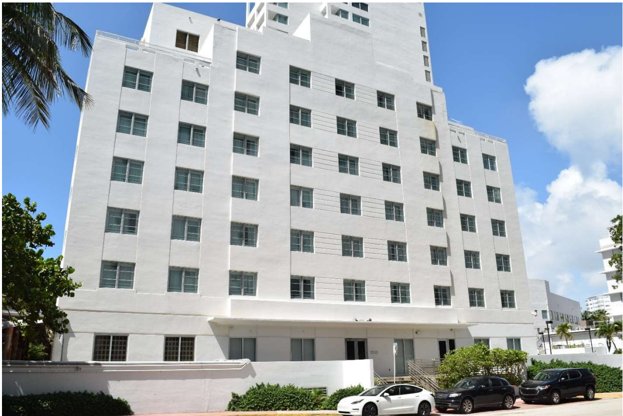
Fig. 188. View of north elevation of former Cromwell Hotel, July 2021.
