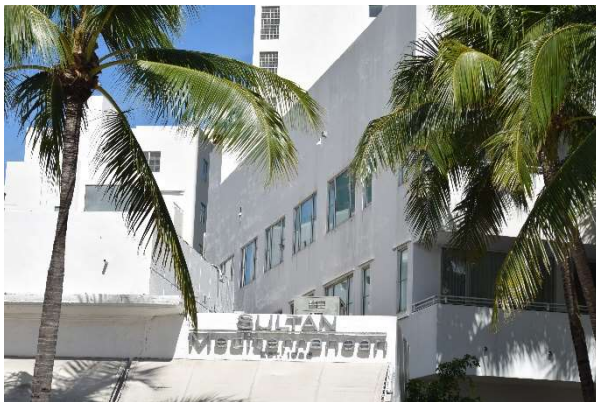
Fig. 159. View of north elevation of Shore Club, looking east, July 2021.
