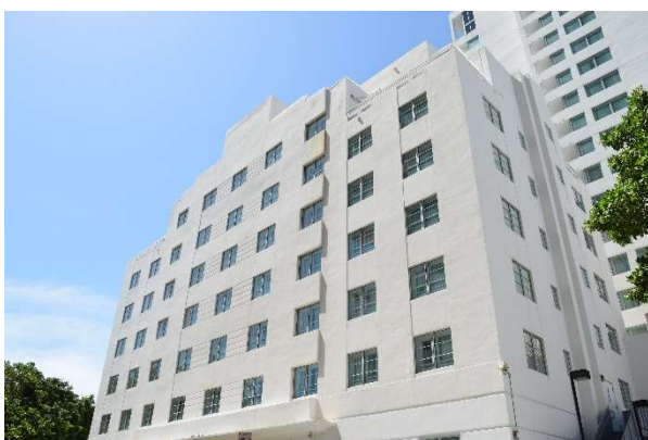
Fig. 189. View of north elevation of former Cromwell Hotel, July 2021.
