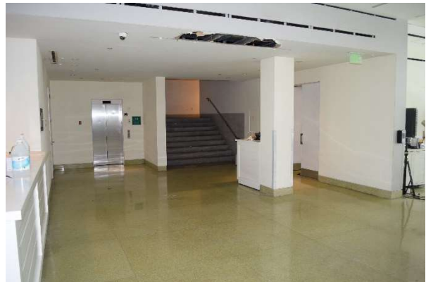
Fig. 170. View of elevator and stair opening at lobby, July 2021
