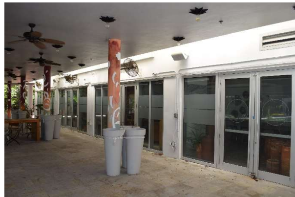
Fig. 198. Detail of storefront at east elevation, July 2021.
