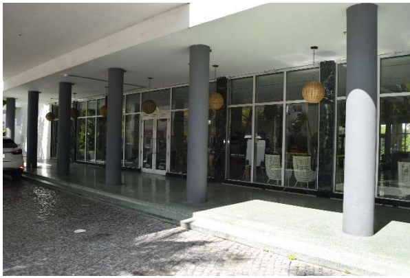
Fig. 152. Detail of entrance canopy at west elevation, July 2021.
