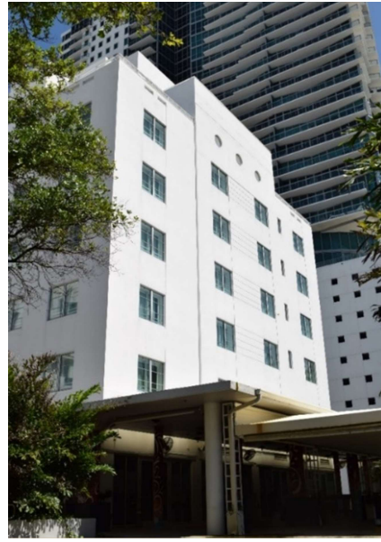
Fig. 196. View of continuous colonnade and attached canopy at east elevation, July 2021.
