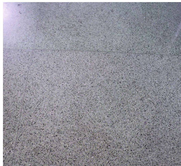
Fig. 155. Detail of terrazzo paving under entrance canopy, July 2021.
