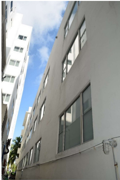
Fig. 167. View of south elevation of Shore Club looking west, July 2021.
