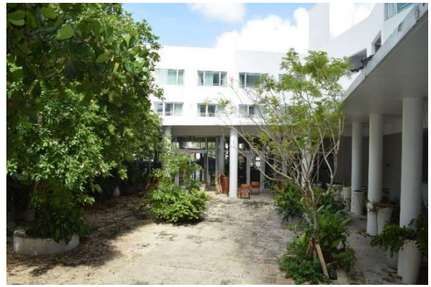
Fig. 166. Detail of wraparound colonnade at courtyard area, July 2021.
