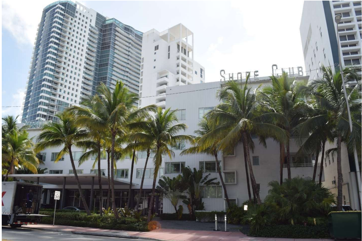
Fig. 146. View of Shore Club Hotel front facade, July 2021.
