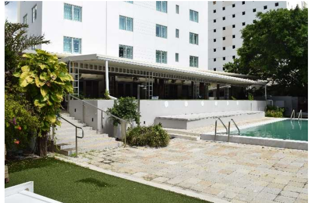
Fig. 137. Detail of canopy at east elevation of Cromwell, July 2021.
