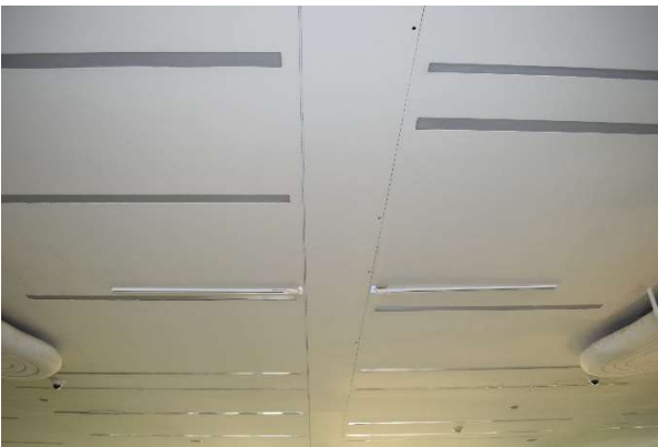
Fig. 175. Detail of ceiling at lobby, July 2021.
