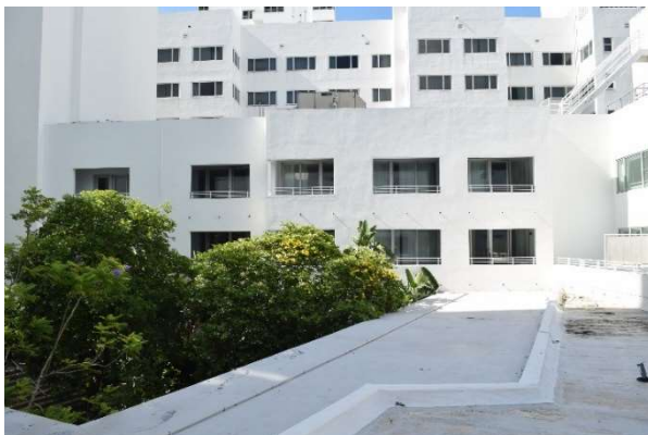
Fig. 163. Detail of recessed balconies at north elevation of south wing, July 2021.
