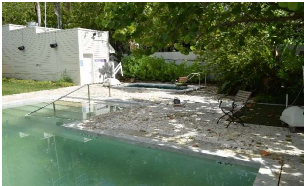
Fig. 144. View of pool equipment building and whirlpool spa, July 2021.
