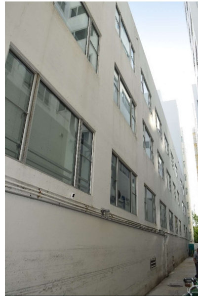
Fig. 168. View of south elevation of Shore Club looking east, July 2021.
