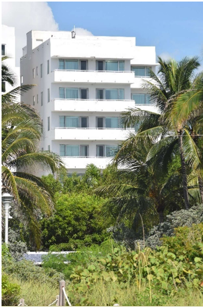
Fig. 182. View of east elevation, looking west, July 2021.
