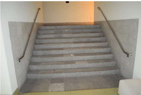
Fig. 177. Detail of Adoquin tile at lobby stairs, July 2021.
