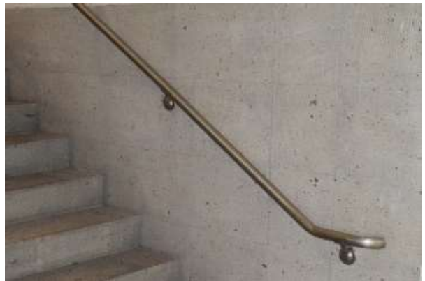
Fig. 178. Detail of handrail at lobby stairs, July 2021.
