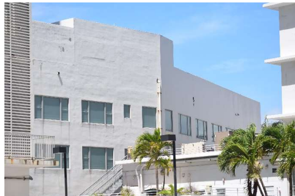
Fig. 160. View of north elevation of Shore Club, looking west, July 2021.
