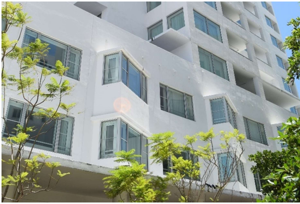
Fig. 165. Detail of angled windows under tower, July 2021.
