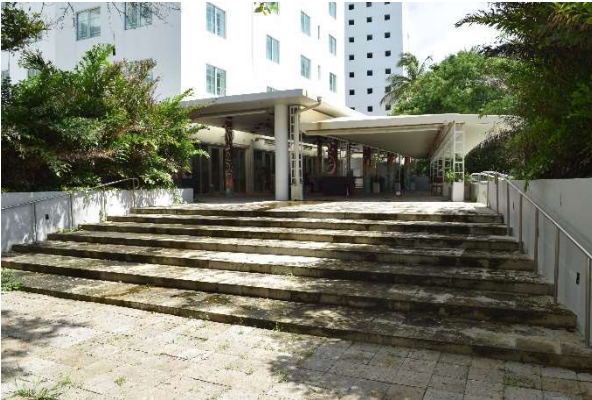
Fig. 136. Detail of stairs from courtyard to Cromwell, July 2021.
