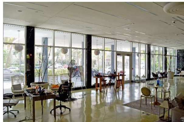
Fig. 172. Detail of marble piers at lobby storefront, July 2021.
