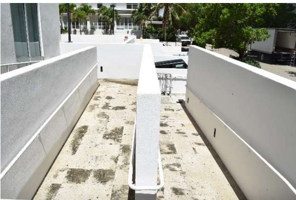
Fig. 127. Detail of accessible ramp at west end of north elevation of Cromwell, July 2021.
