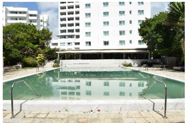
Fig. 139. View of main pool looking west toward Cromwell, July 2021.
