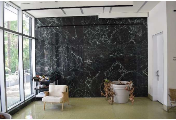
Fig. 173. Detail of marble wall and base at lobby, July 2021.
