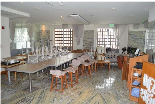
Fig. 5. Detail of marble flooring and wainscot at restaurant space, July 2021.
