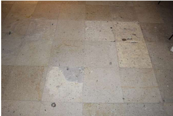
Fig. 3. Detail of flooring in lobby, July 2021.
