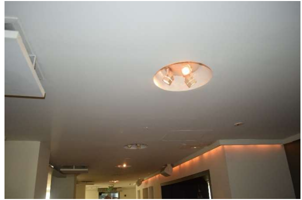
Fig. 4. Detail of ceiling finish and recessed light fixture at lobby, July 2021.
