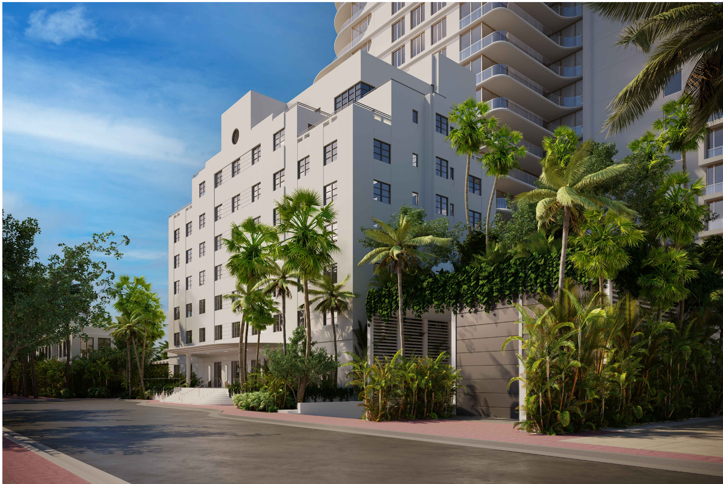
VIEW FROM 20th STREET AT THE SERVICE BUILDING
