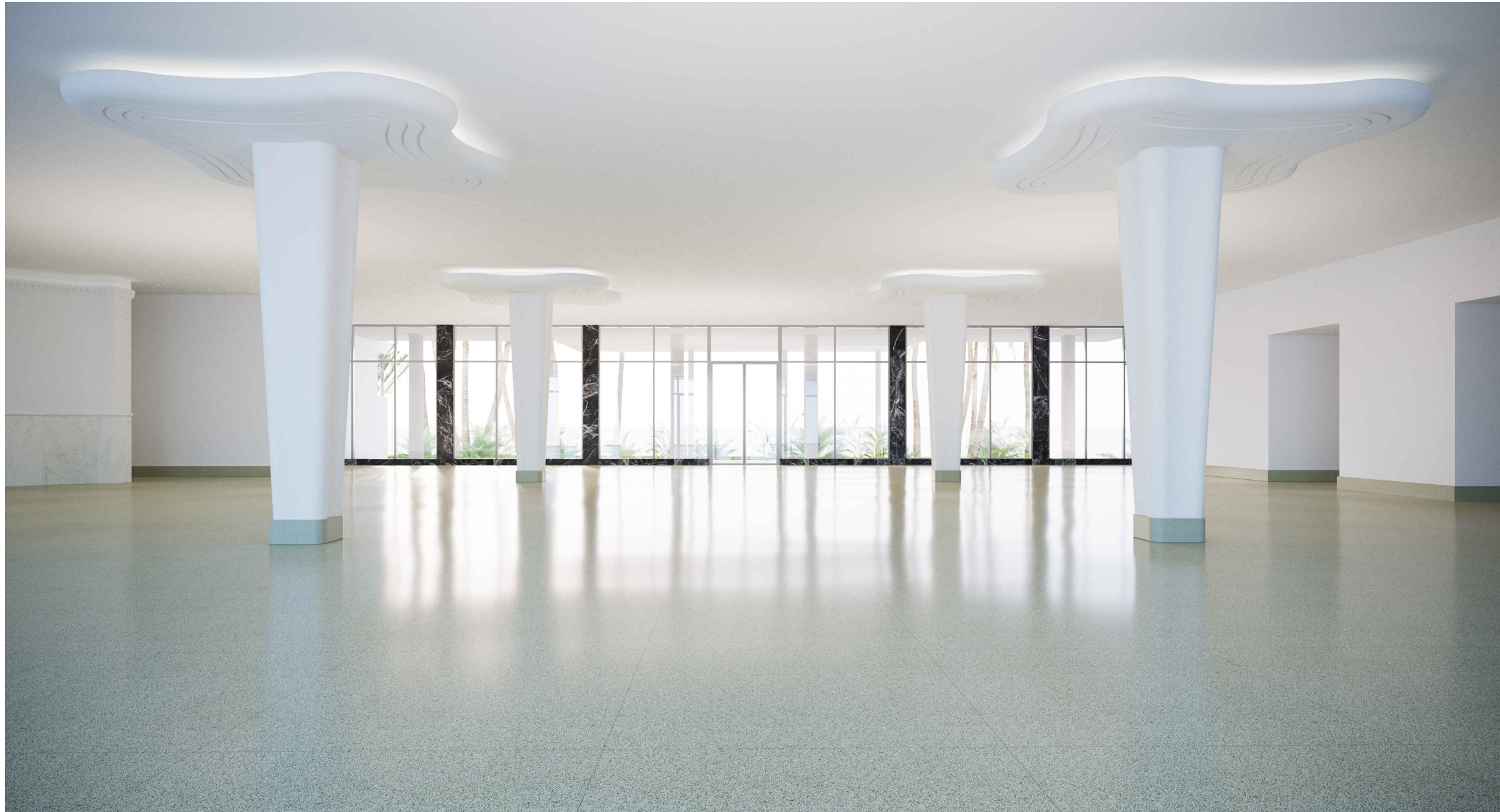
SHORE CLUB LOBBY FACING WEST
