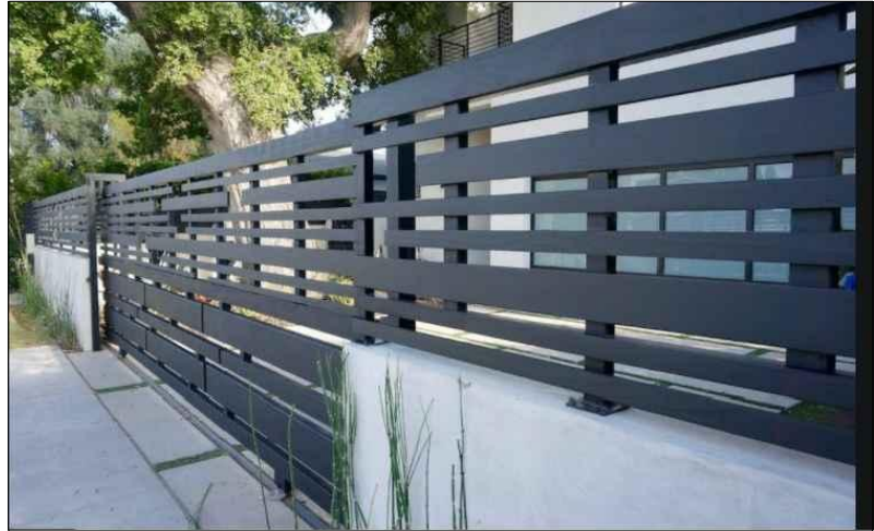
ALUMINUM GATE AND FENCE ABOVE RETAINING WALL
