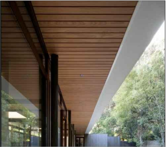
WOOD CEILING UNDER ROOF OVERHANGS
