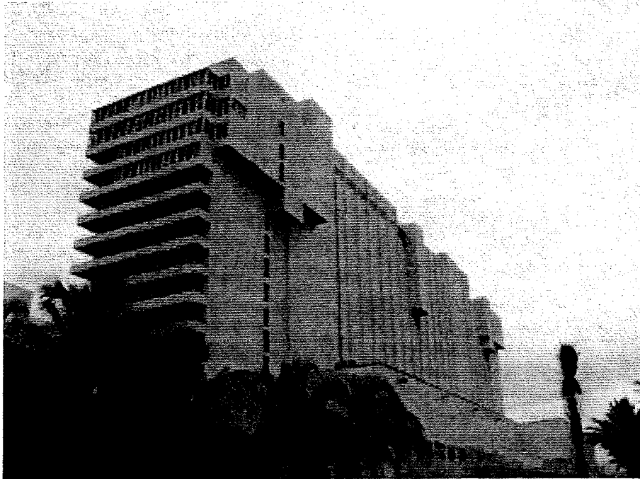
North wall of Versailles Tower from boardwalk ATS photo 2005
