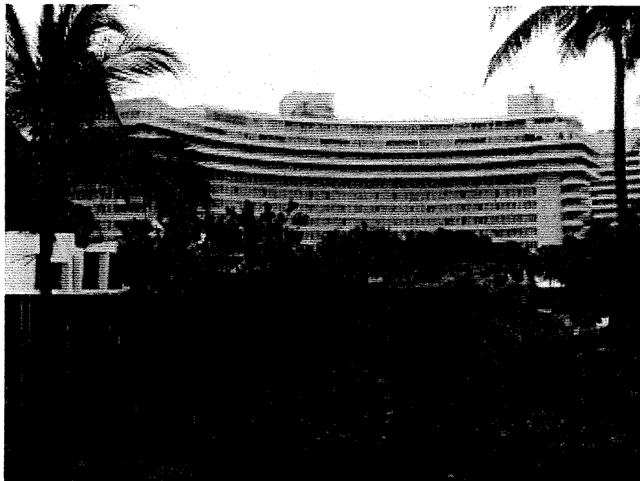
View of Chateau from boardwalk southeast ATS photo 2005
