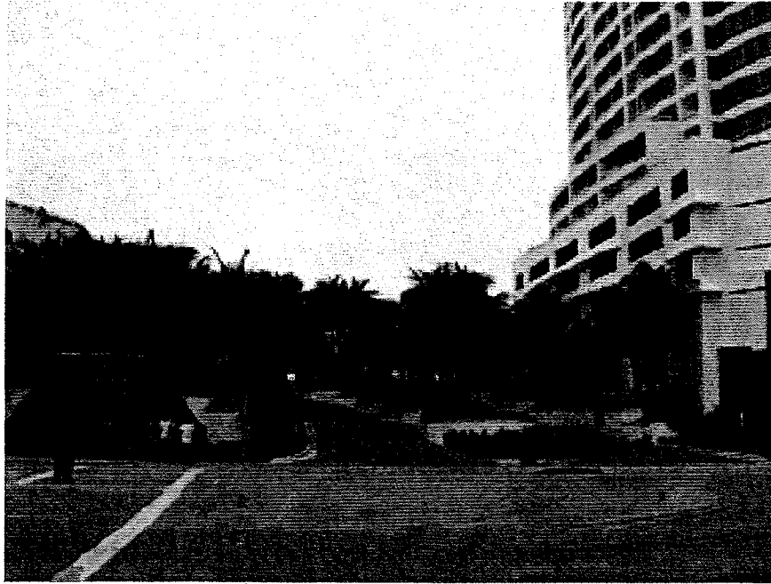
New Entrance from Collins Avenue ATS photo 2005
