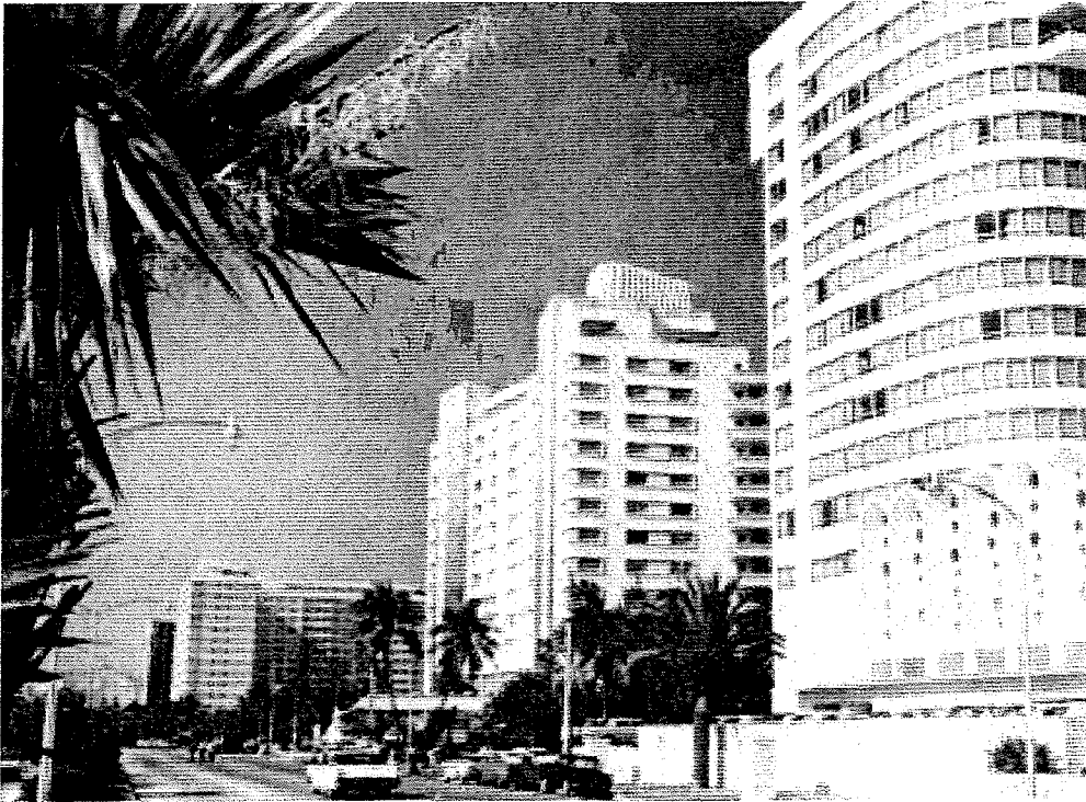
Collins Avenue looking North: View of North Tower & "Cheese Wall" with Eden Roc Beyond Image Courtesy of the Florida Photographic Collection
