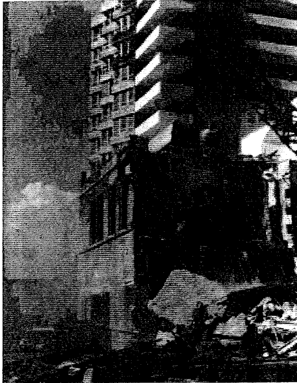
Demolition of Firestone Mansion Image Courtesy of the Historical Museum of South Florida, Miami News Archives
