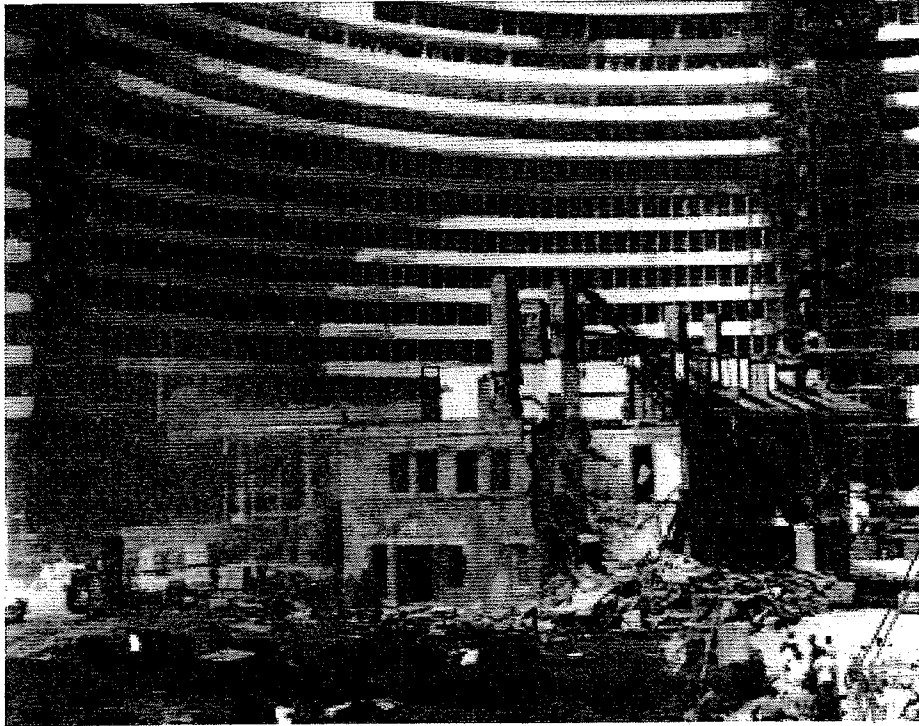
Demolition of Firestone Mansion Image Courtesy of the Historical Museum of South Florida, Miami News Archives
