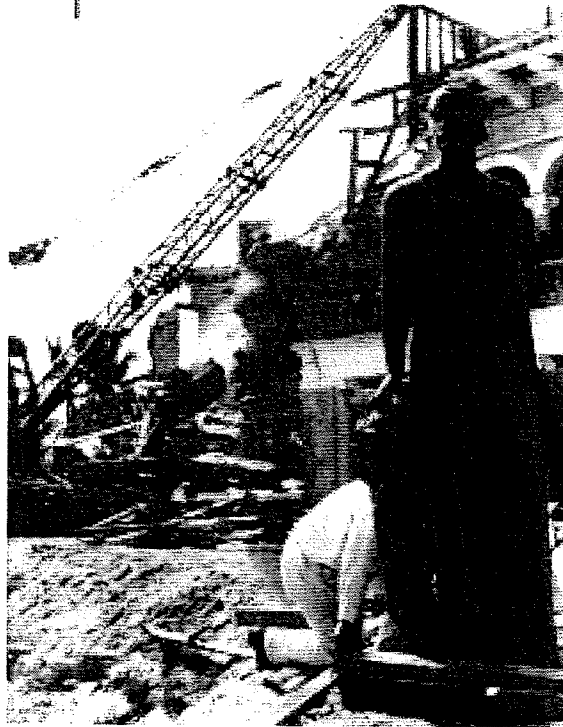
Demolition of Firestone Mansion Image Courtesy of the Historical Museum of South Florida, Miami News Archives
