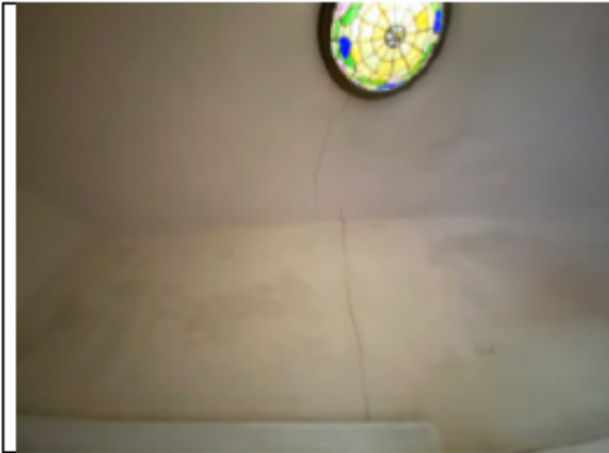
Photo 19 – 2 nd floor wall plaster cracking due to settlement
