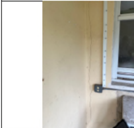
Photo 3 - Wall cracking on East elevation
