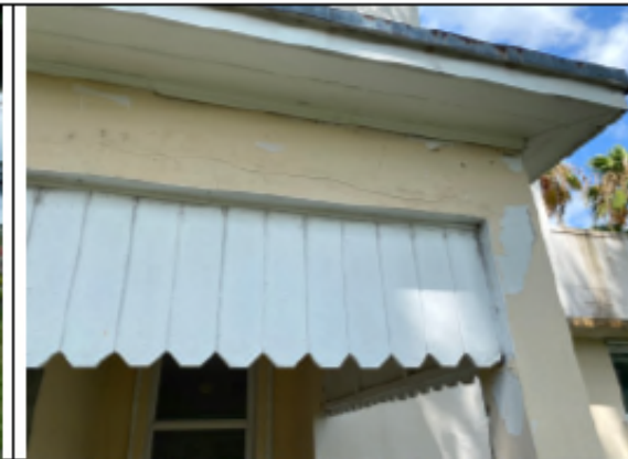
Photo 2- Concrete beam cracking in back of garage
