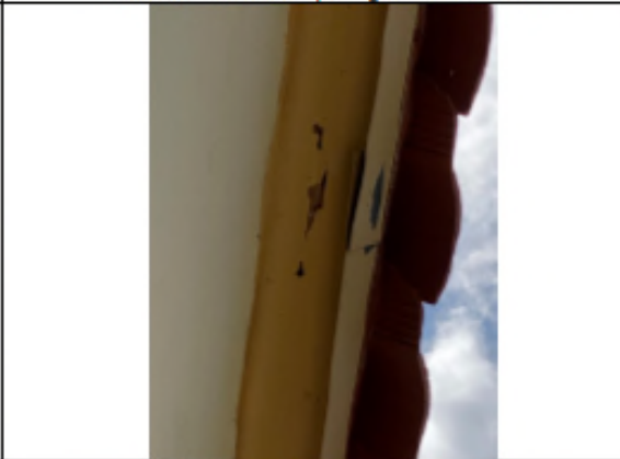
Photo 12 – Roof eave termite damage
