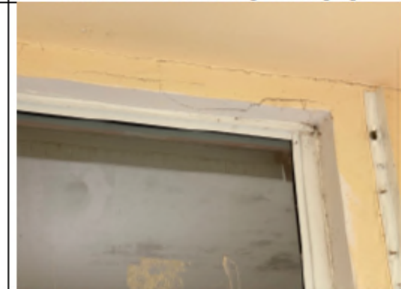
Photo 4 - Beam cracking over window on East elevation
