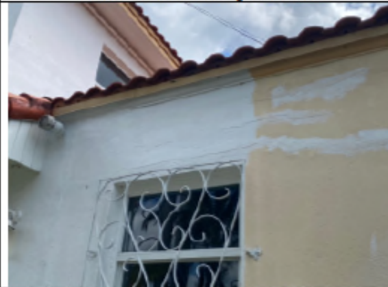
Photo 11 - West Elevation, concrete spalling
