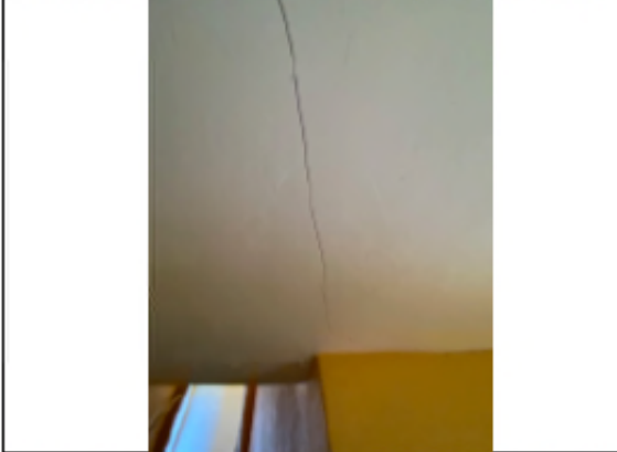
Photo 21 - 2 nd floor ceiling plaster cracking due to settlement
