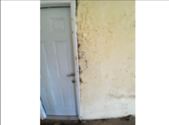
Photo 24 – Moisture damage on walls
