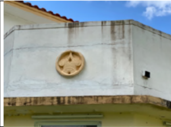
Photo 7 - North East Elevation wall and beam cracking
