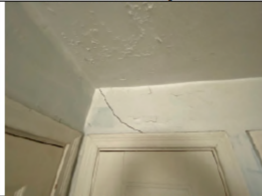
Photo 17 – Plaster cracking over door indicative of settlement
