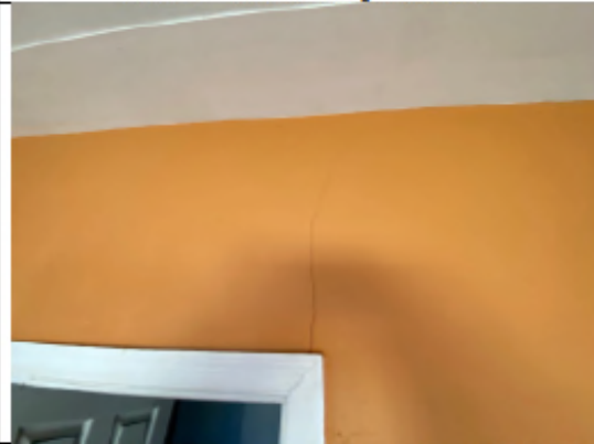
Photo 16 – Plaster cracking over door Indicative of settlement
