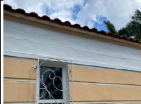
Photo 10 – Concrete spalling on SW elevation
