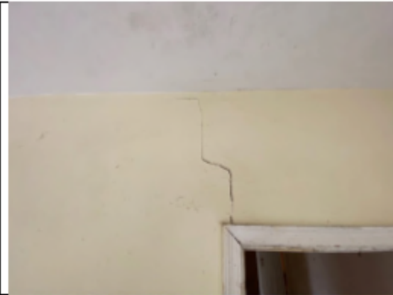
Photo 20 – 2 nd floor wall plaster cracking due to settlement
