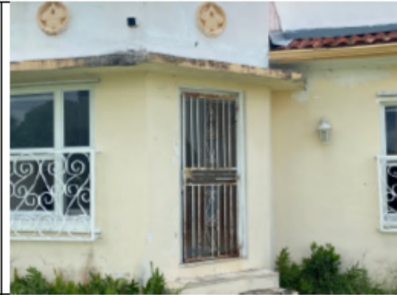
Photo 8 – NW corner beam cracking over eyebrow
