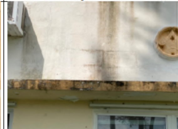
Photo 6 - Drop in office (South west corner) due to foundation settlement
