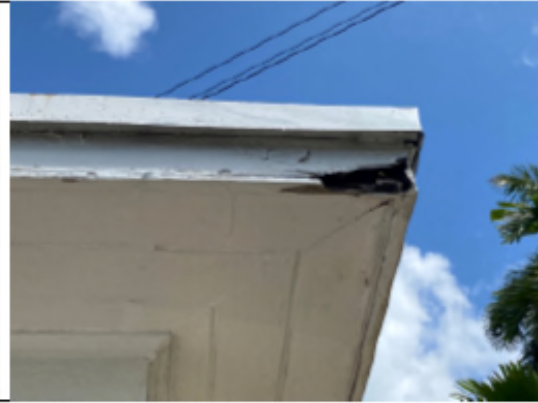
Photo 13 – SE Elevation, roof Eave damage
