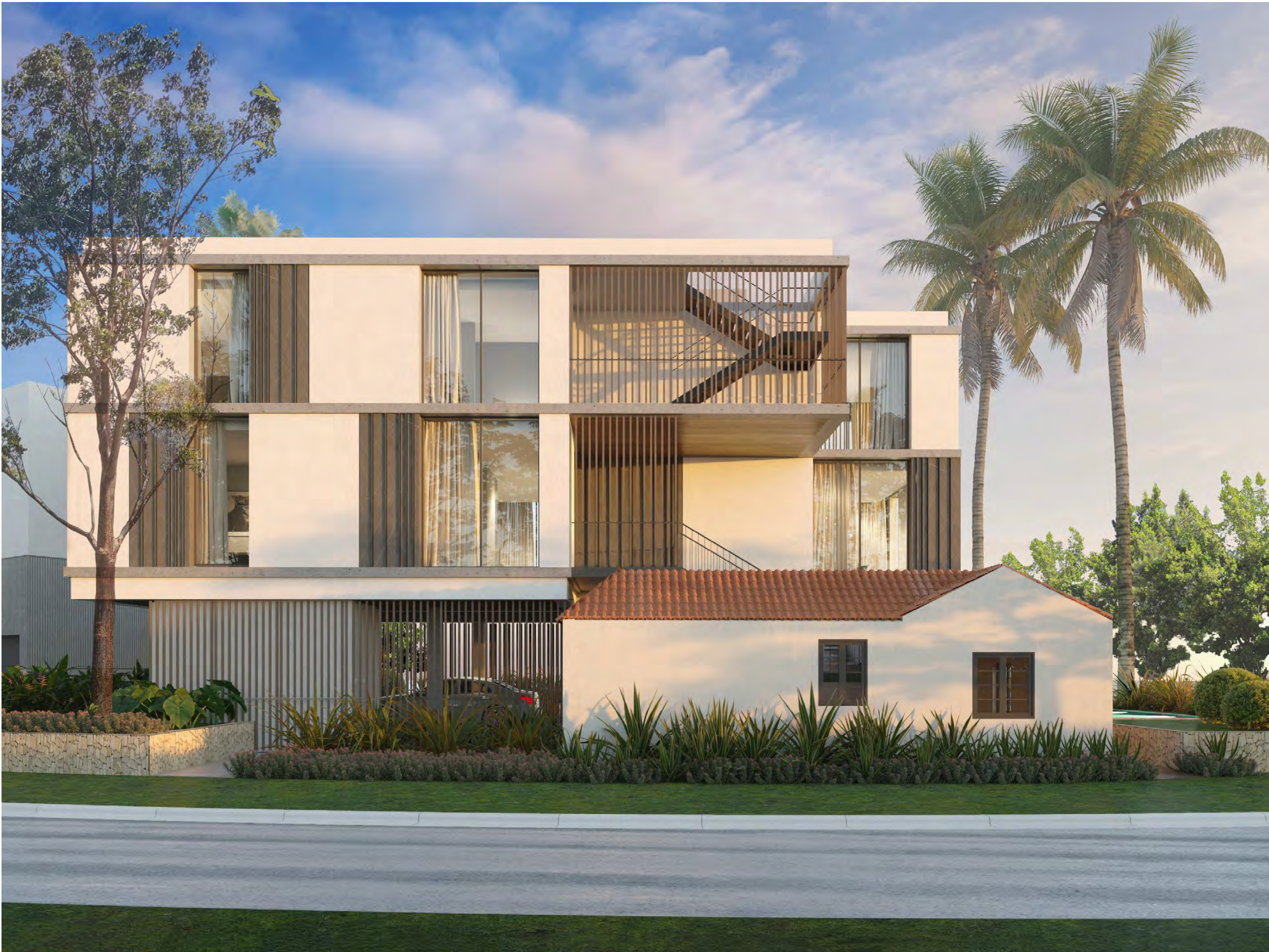
VIEW FROM NORTH COCONUT LANE
