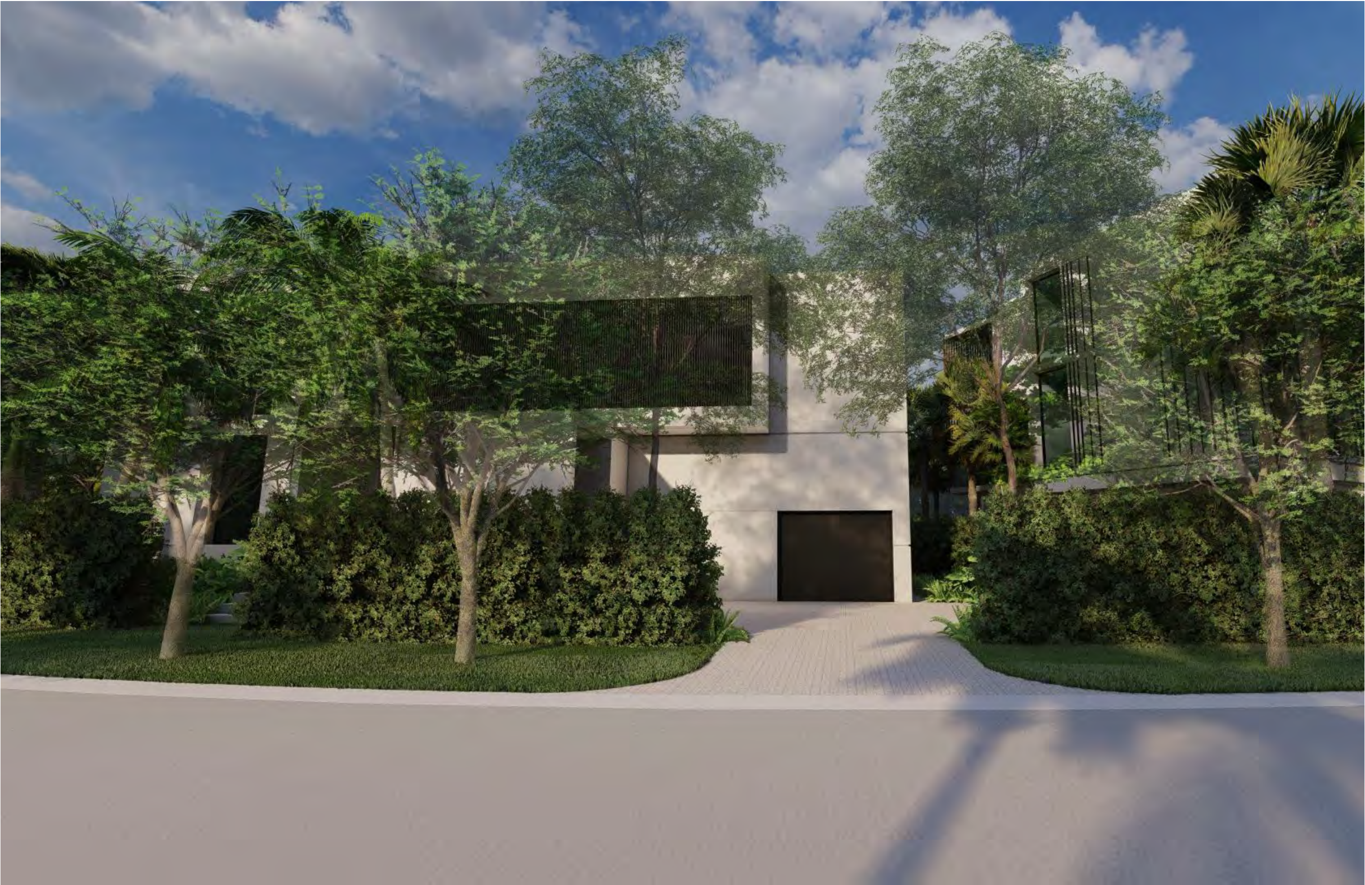
VIEW FROM NORTH COCONUT LANE
