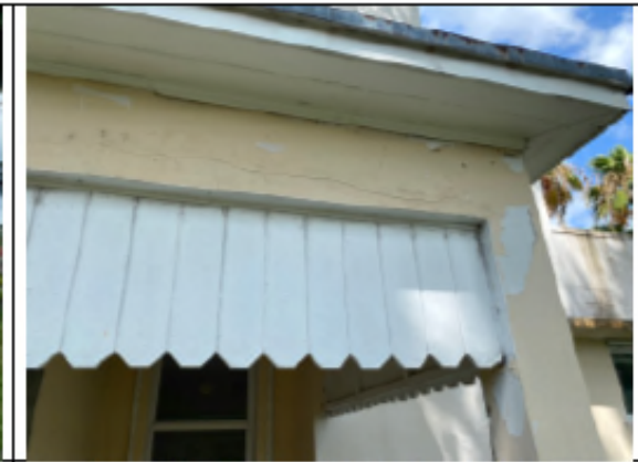
Photo 2- Concrete beam cracking in back of garage
