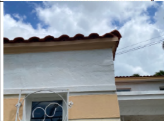
Photo 9 - Concrete Cracking SW elevation
