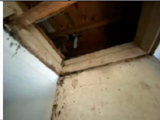
Photo 18 – Wood Damage of 2 nd floor
