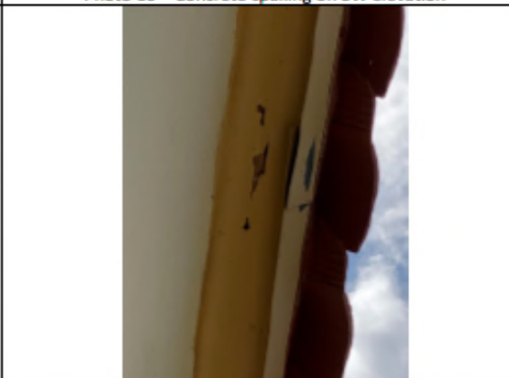
Photo 12 – Roof eave termite damage
