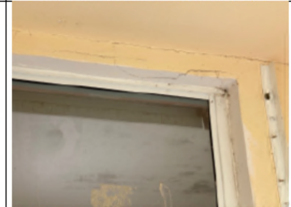
Photo 4 - Beam cracking over window on East elevation
