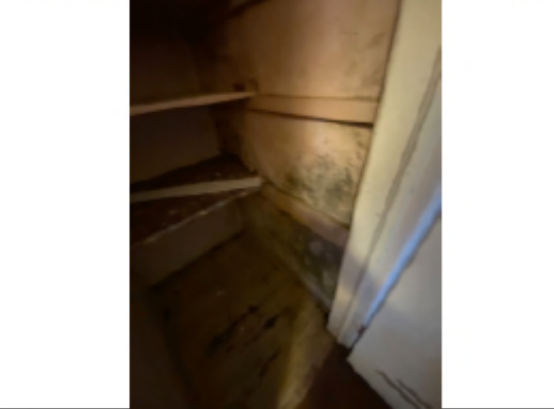
Photo 22 – mold presence in the second floor
