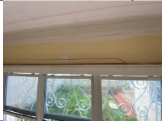
Photo 15 – SE Elevation cracking over window
