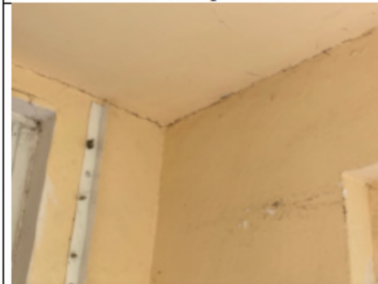
Photo 5- wall / roof separation on East elevation foundation settlement
