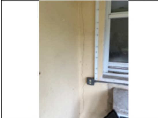
Photo 3 - Wall cracking on East elevation
