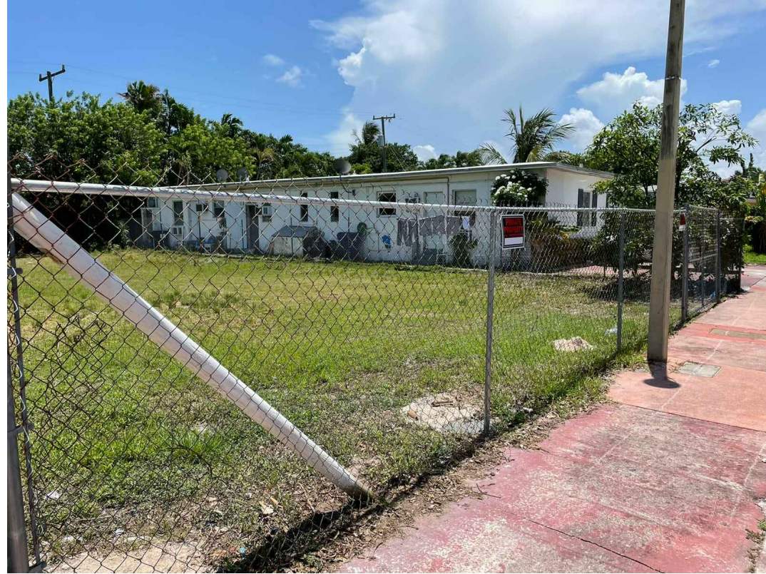
SITE VIEW LOOKING SW FROM 84 STREET
