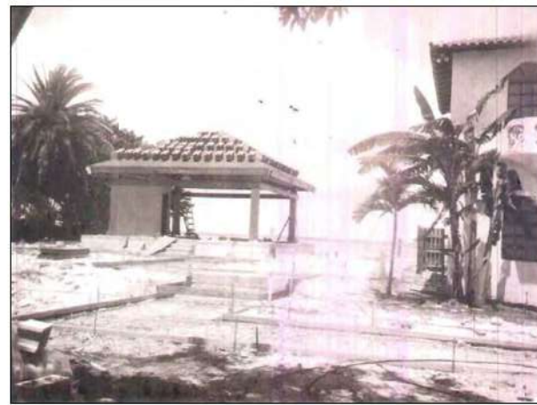
2 1985 PHOTO OF CABANA UNDER CONSTRUCTION Scale: N.T.S
