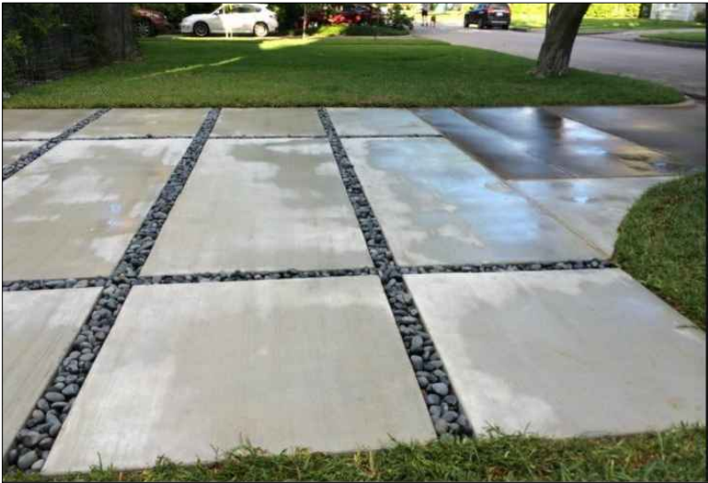
DRIVEWAY: CONCRETE WITH RIVER ROCK INSERTS
