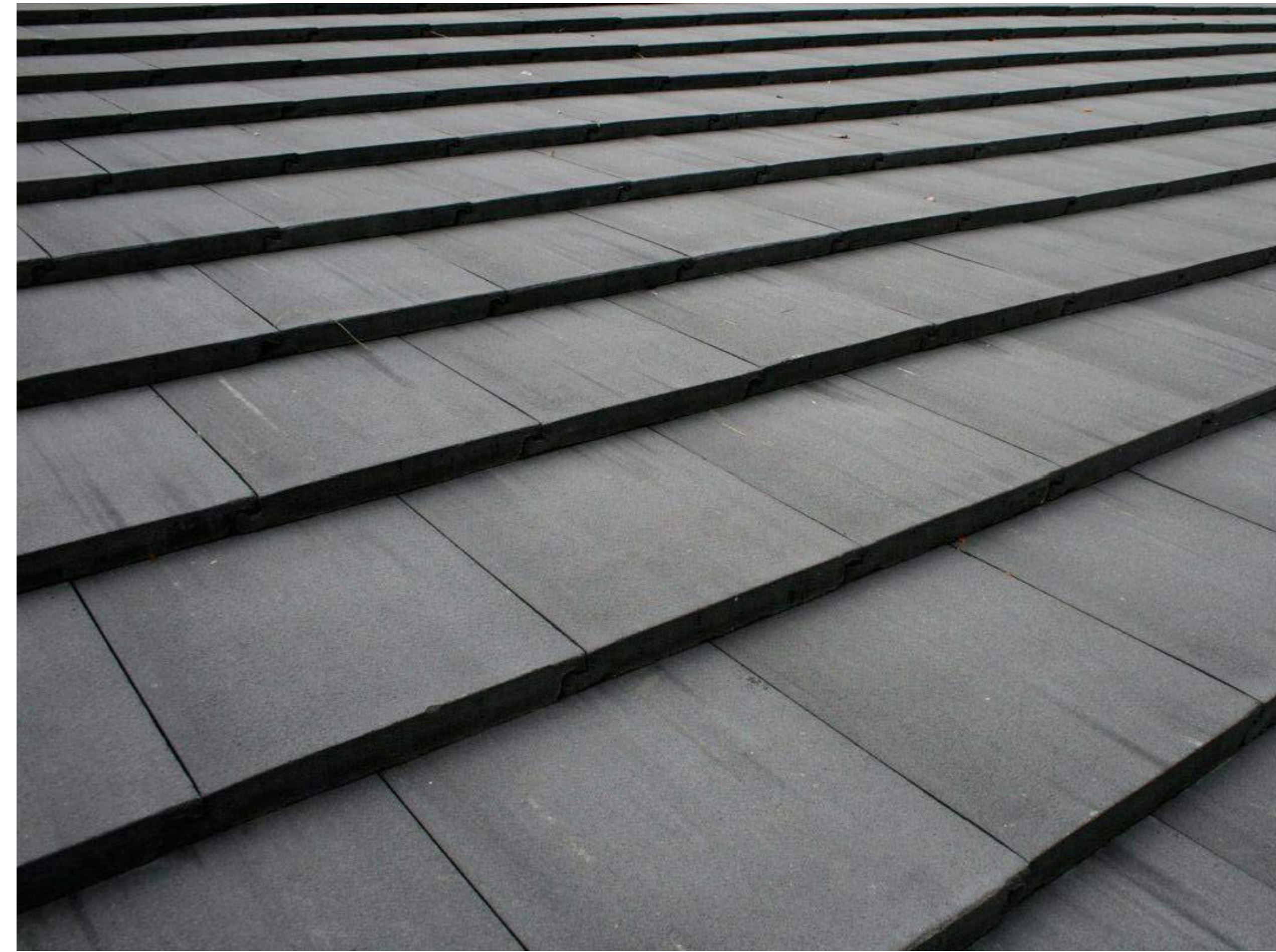
CONCRETE ROOF TILES
