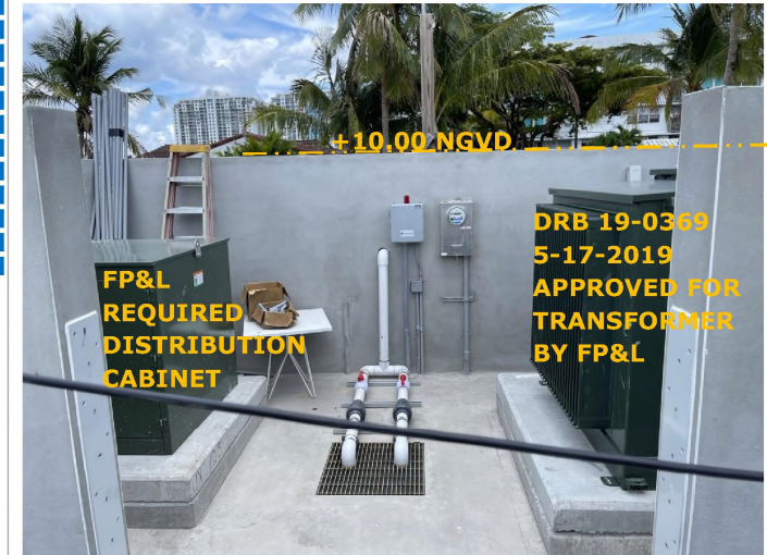
FP&L TRANSFORMER + DISTRIBUTION CABINET WEST VIEW
