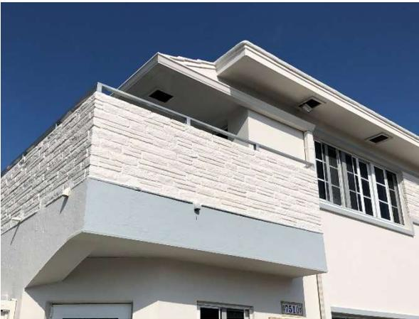
*Fig. 39. Detail of overhanging upper walkway and stone veneer, March 2021.*
