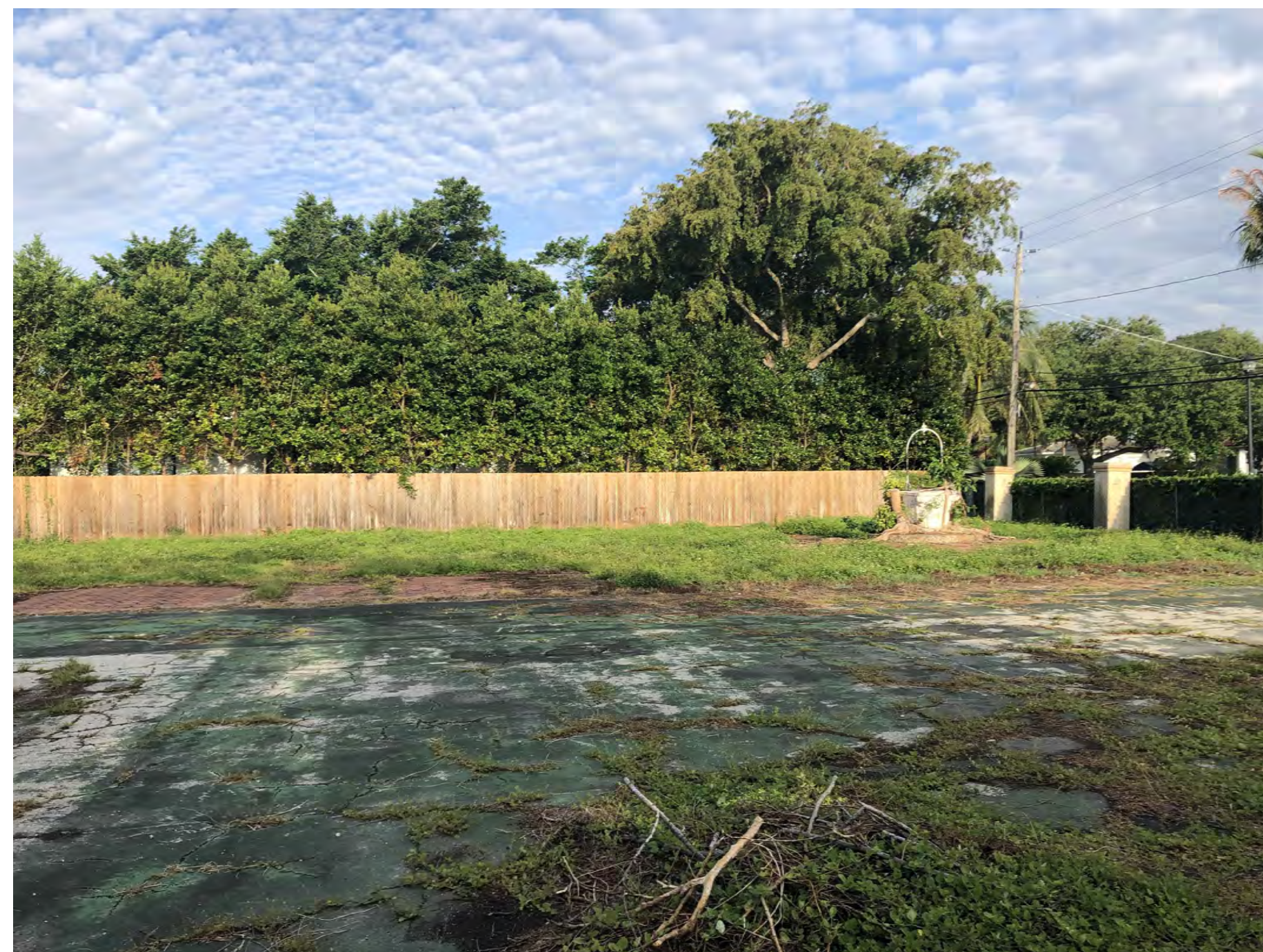
E3 - 420 W 51ST ST VIEW TO WEST SIDE
