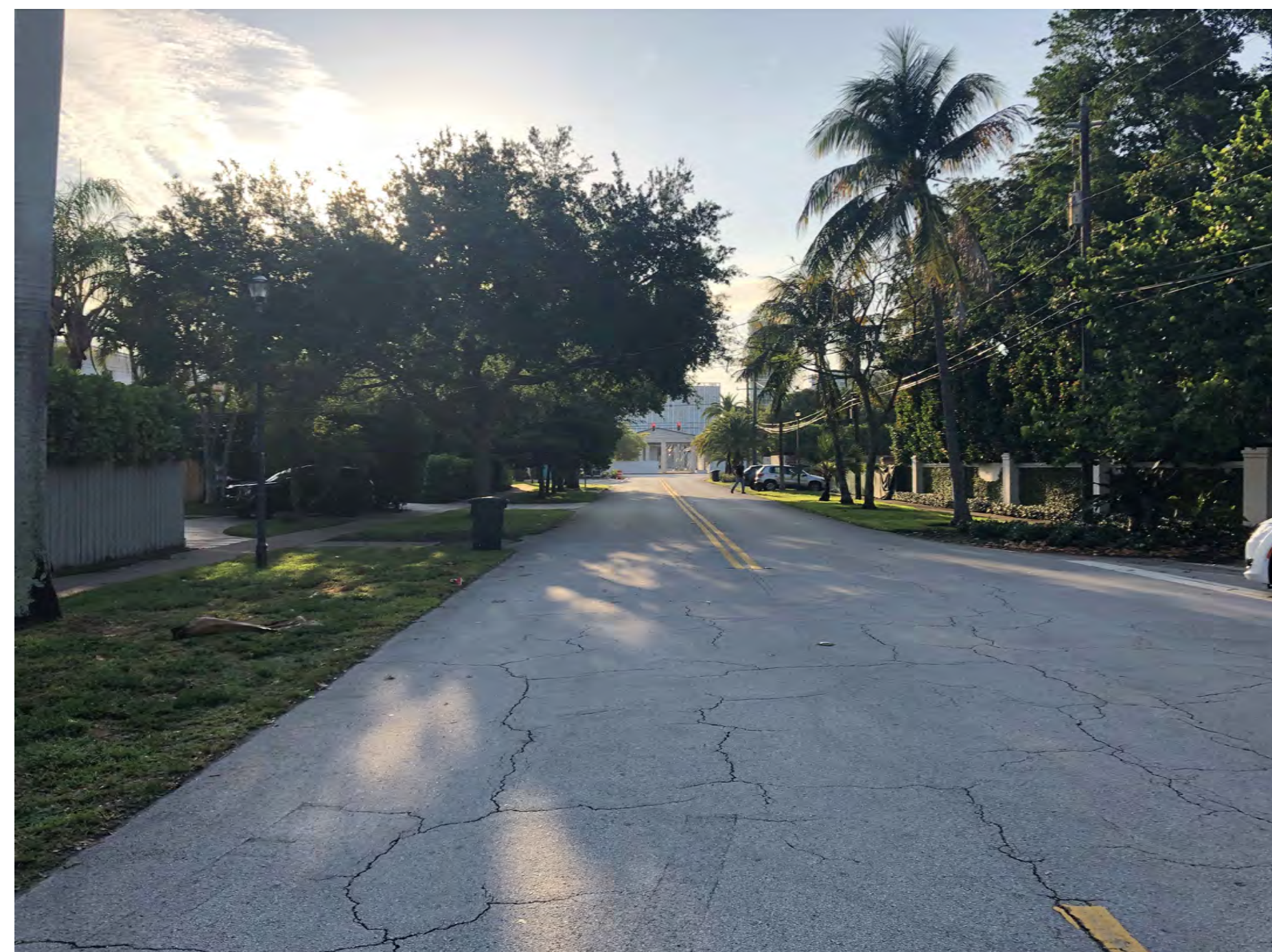
C1 - W 51ST ST (VIEW TO EAST)
