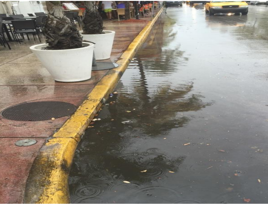
Figure 3: Grates clog and backup water into the street.
