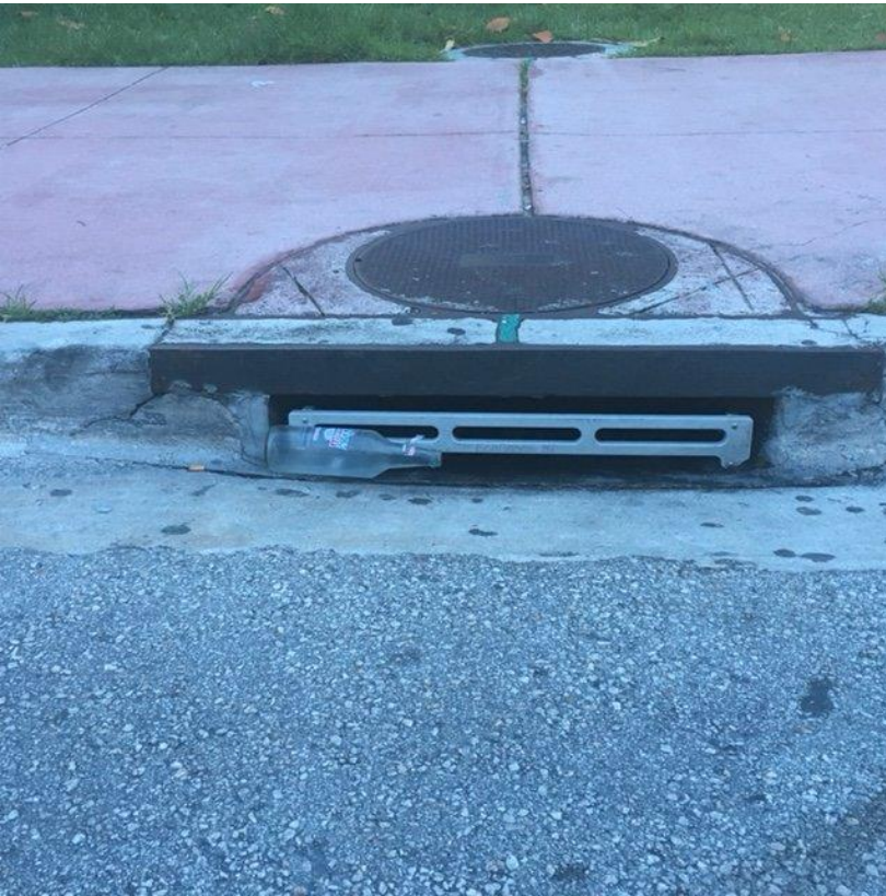
Figure 4: EcoSense grates are better for stopping larger items but need to be cleaned frequently by street sweepers.
