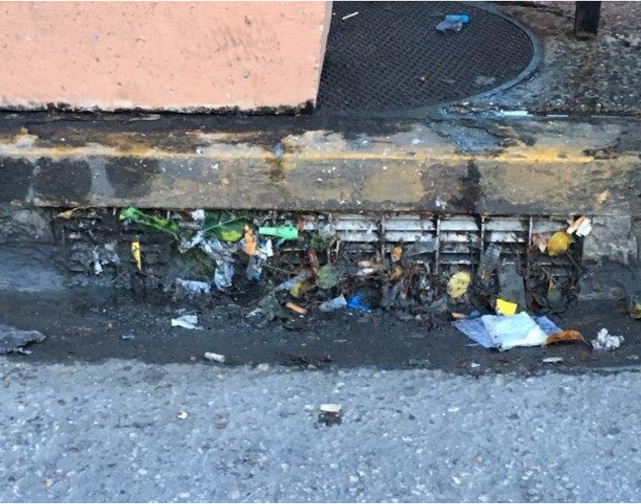
Figure 2: Stop Ocean Pollution Grates clogged with trash and debris do not look aesthetically pleasing in between cleanings.
