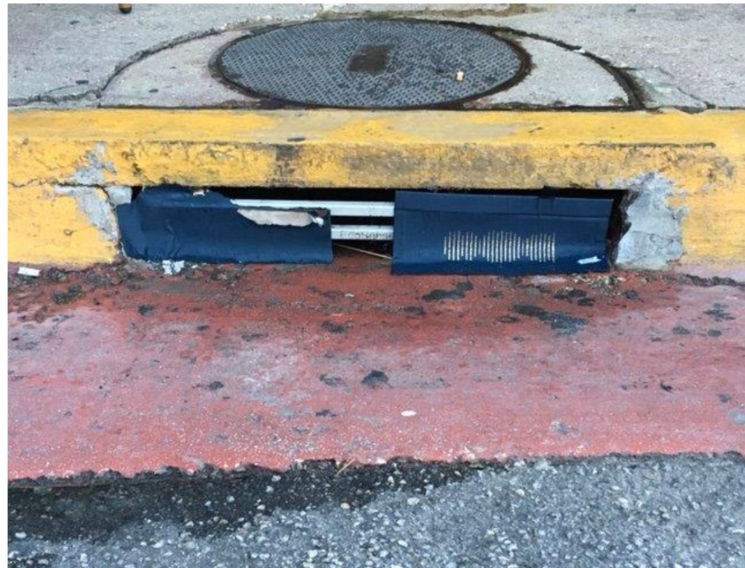
Figure 4: EcoSense grates are better for stopping larger items but need to be cleaned frequently by street sweepers.
