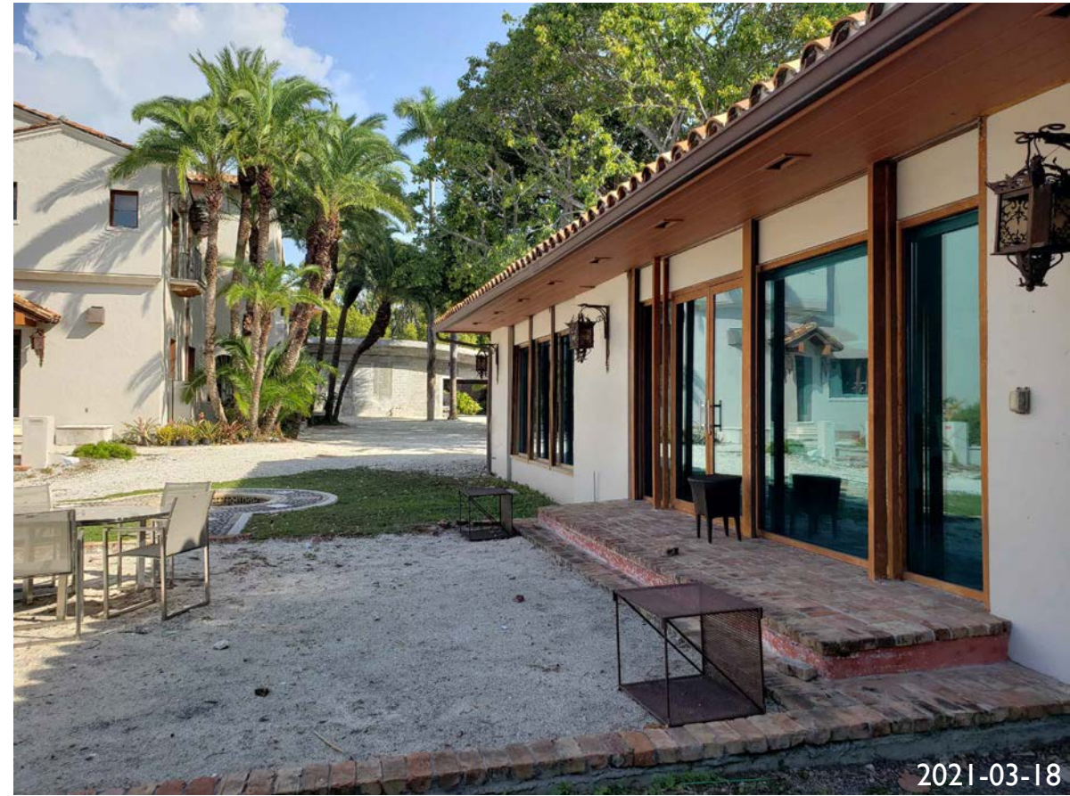
6. VIEW OF LOT 4 FACING NORTH
