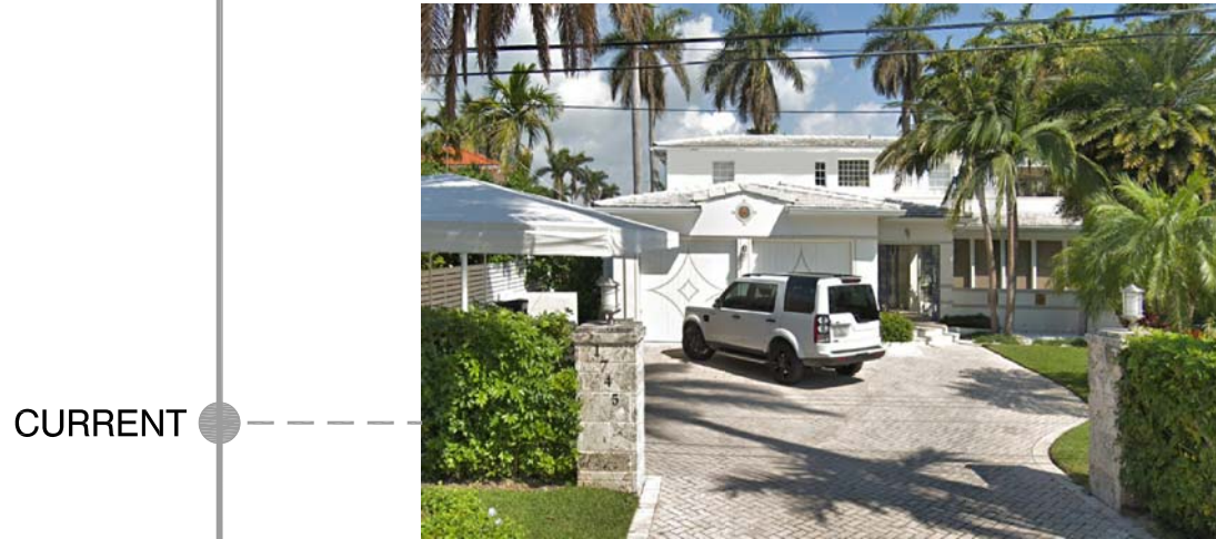
05 CURRENT FRONT PHOTOGRAPH
