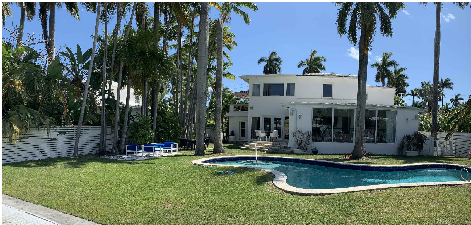
02 NORTH FACADE (REAR VIEW)
