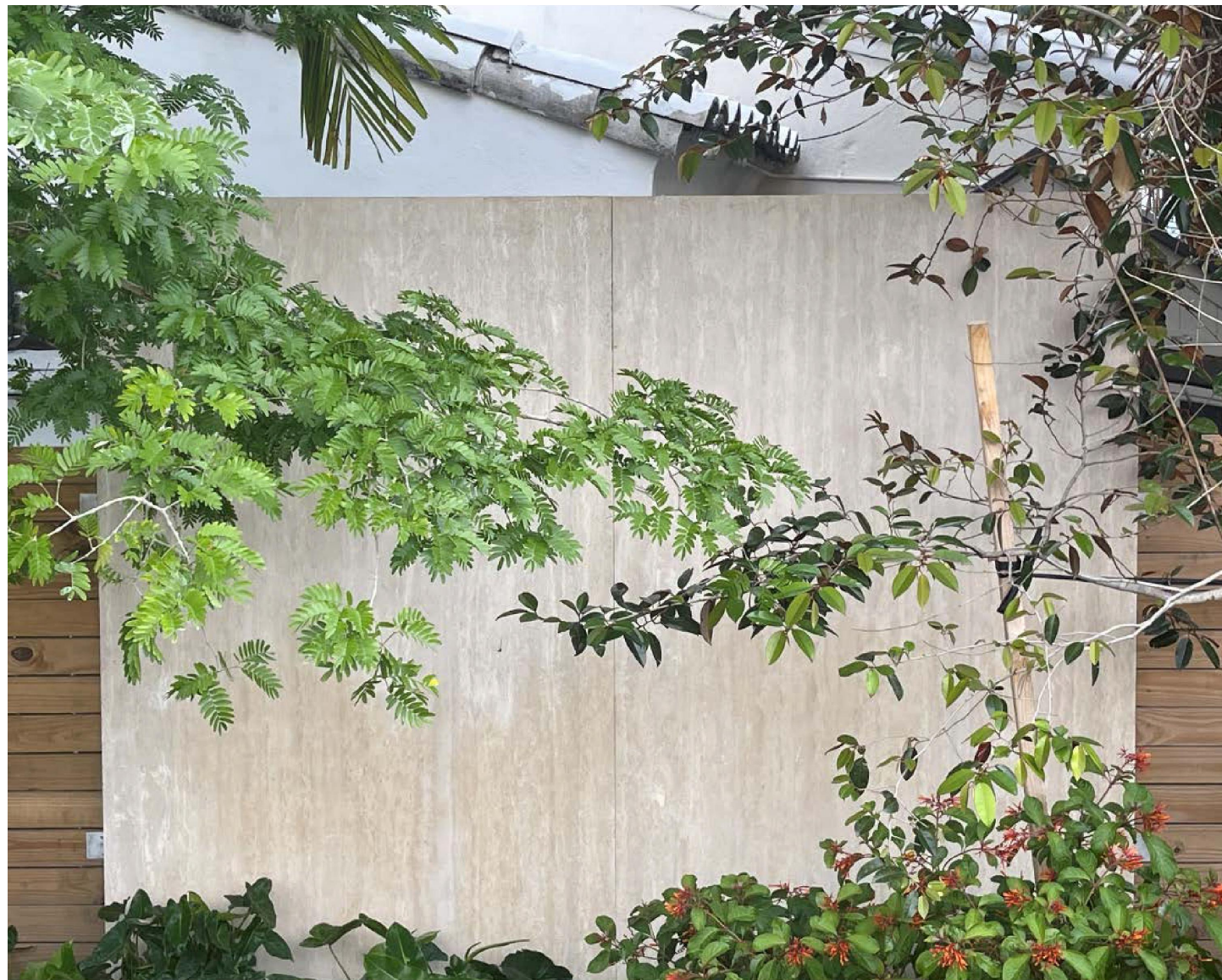
TRAVERTINE STONE CLADDING MOCKUP
