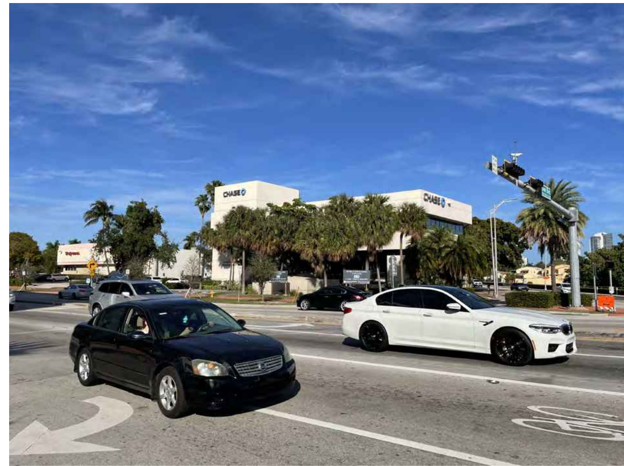
02 ALTON ROAD / DADE BLVD LOOKING NORTH EAST AT 1801 ALTON ROAD
