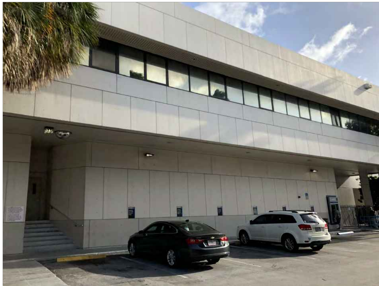
09 EXISTING PARKING LOOKING SOUTHWEST
