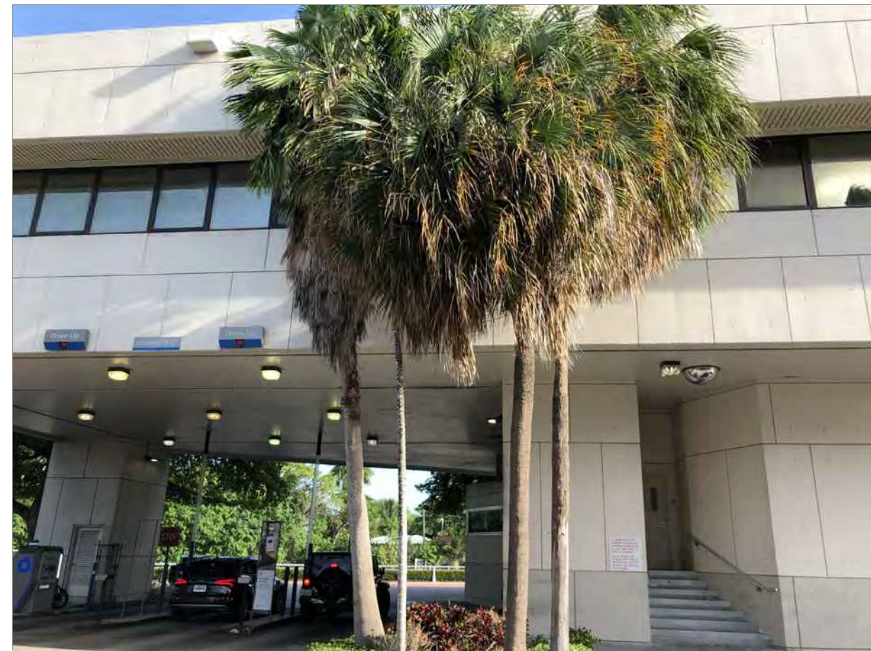
10 EXISTING PARKING LOOKING SOUTH
