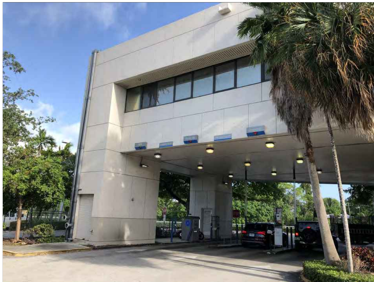
11 EXISTING PARKING LOOKING SOUTHEAST
