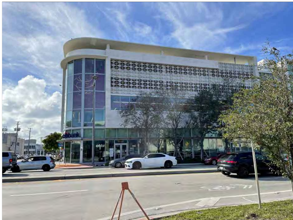
19 ALTON RD / DADE BLVD LOOKING WEST AT MICHAEL'S BUILDING
