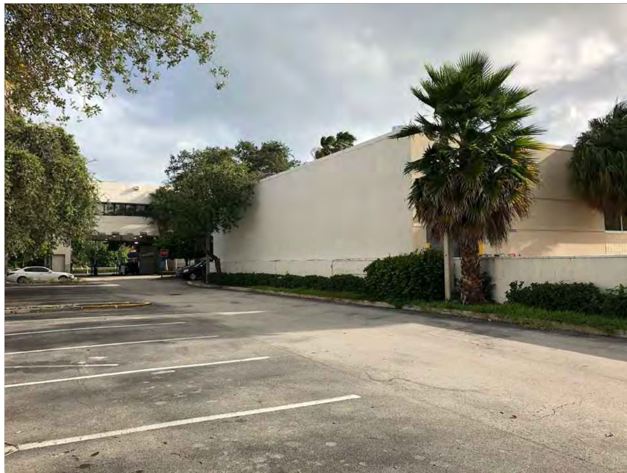
13 EXISTING PARKING LOOKING SW
