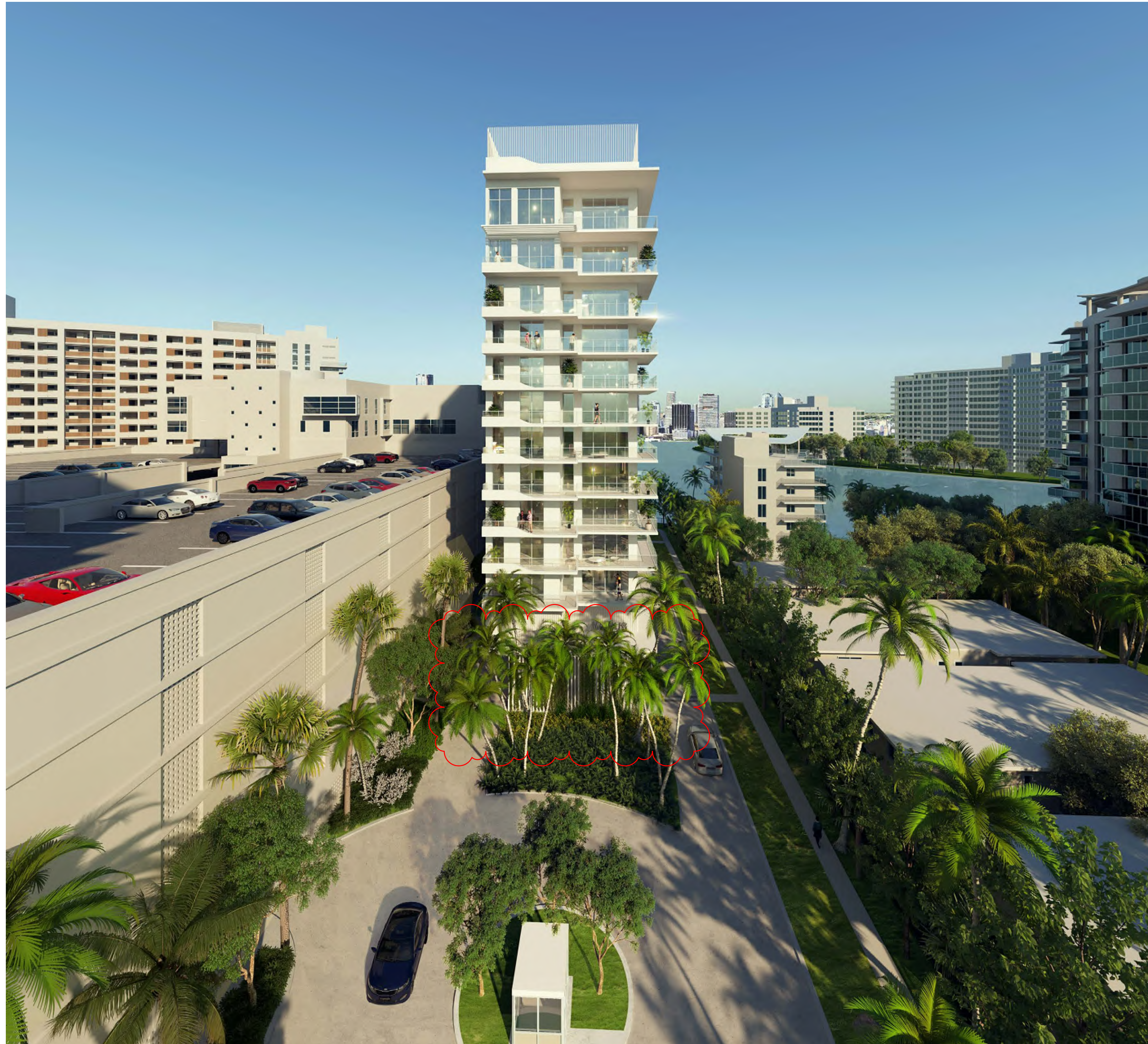
VIEW FROM BAY ROAD - FACING WEST
