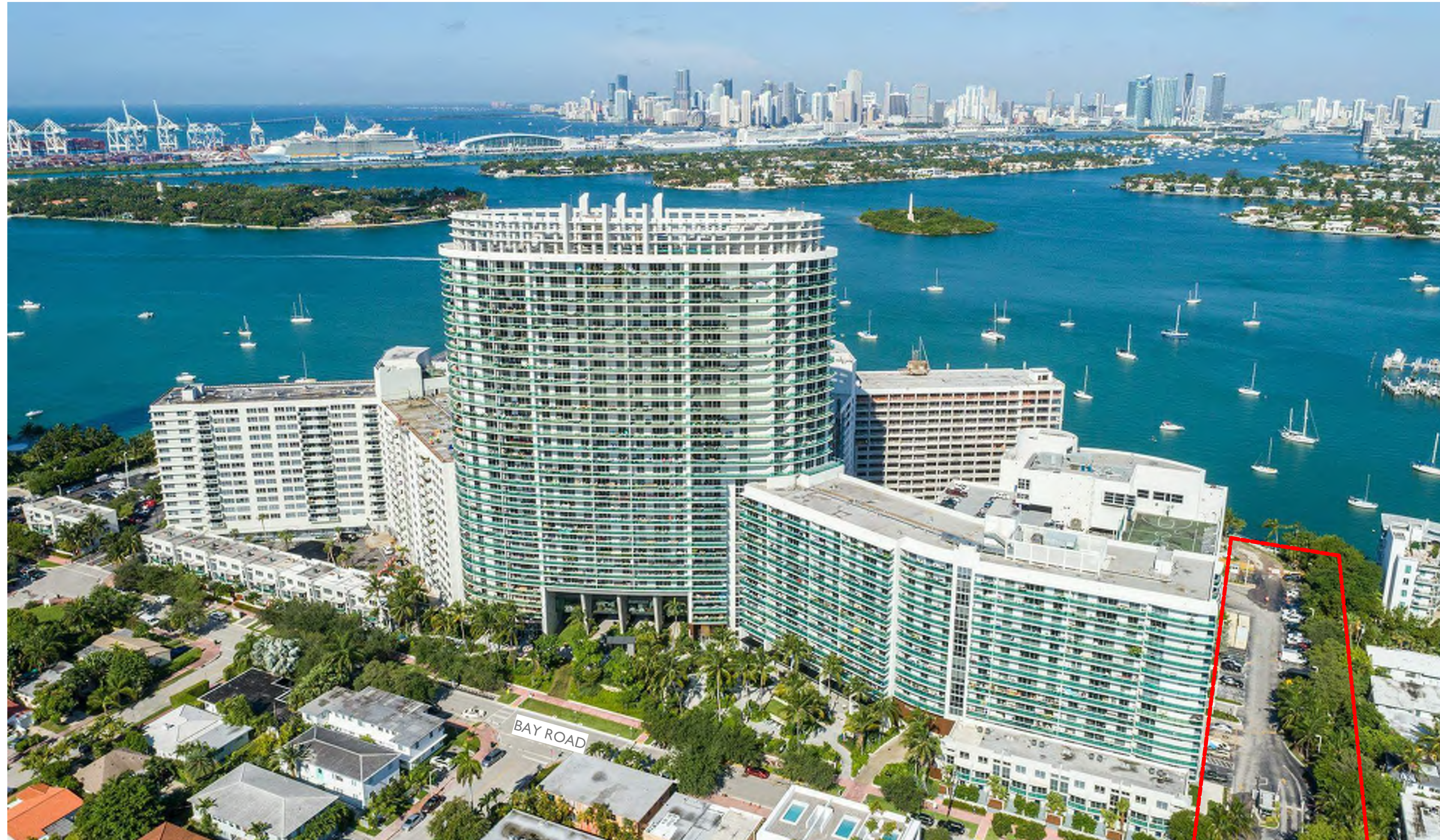
NEW TOWER SITE
