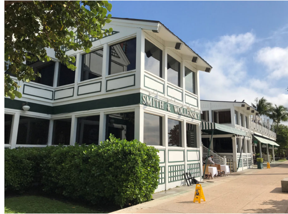
Photo 2 – Rear Elevation from Bay Walk
