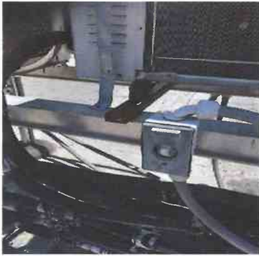
8 1 - Closet/Utility/Mechanical Outlets/Switches - Missing outlet cover on roof top
