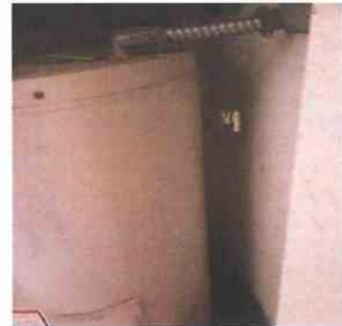
18 1 Unit 1-106 - Local Systems Water Heater - Missing pressure release tube
