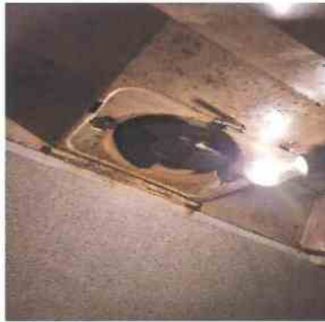
14 1 Unit 1-105 - Kitchen Range Hood/Vent Fan - Missing cover
