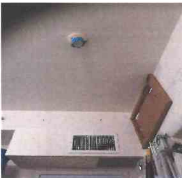
24 1 - Office Smoke Detector - Smoke detector to fire department covered
