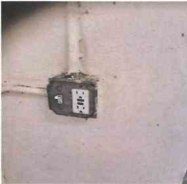
18 1 - Closet/Utility/Mechanical Outlets/Switches - GFCI in elevator room non op
