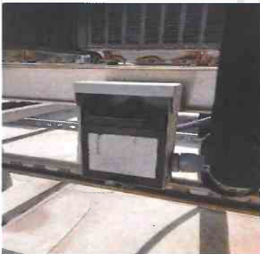
4 1 - Closet/Utility/Mechanical Electric Panel - Missing cover on roof top
