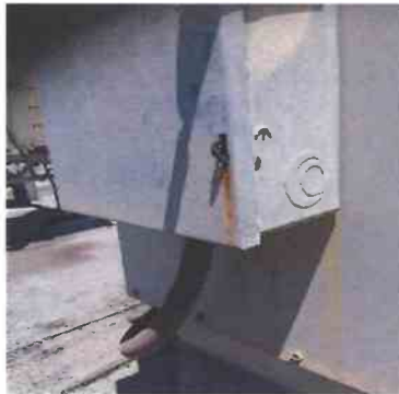
12 1 - Other Community Spaces HVAC System - HVAC on roof handel not secured.
