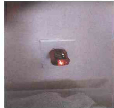
31 1 Unit 1-207 - Bedroom 1 Outlets/Switches - Open ground
