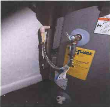
11 1 Unit 1-5 - Local Systems Water Heater - Improperly installed
