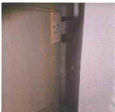
22 1 Unit 1-203 - Local Systems Water Heater - Missing pressure release tube
