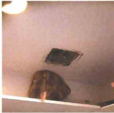
11 1 Unit 1-105 - Bathroom 1 Ventilation/Exhaust - Missing vent cover
