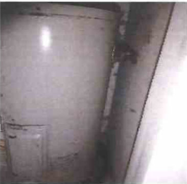
16 1 Unit 1-105 - Local Systems Water Heater - Missing pressure release tube, needs to be within 6 in
