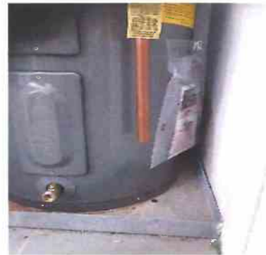
13 1 Unit 1-502 - Local Systems Water Heater - Tube needs to be within 6 inches of floor
