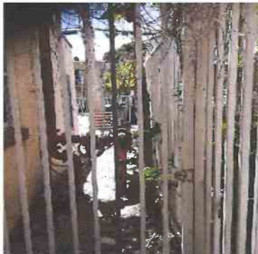
7 1 - Entry Door Door - Security/Storm - Right side of building will not open
