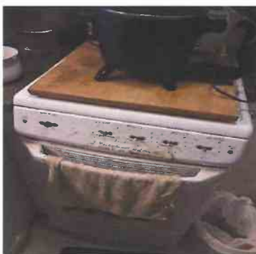
26 1 Unit 1-206 - Kitchen Stove/Range - Missing stove knobs
