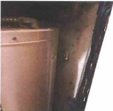
34 1 Unit 1-302 - Local Systems Water Heater - Missing pressure release tube
