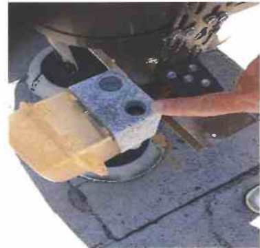
13 1 - Other Community Spaces Outlets/Switches - Missingcover on rooftop HVAC junction box.
