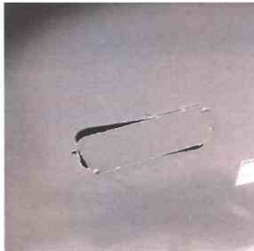
22 1 - Local Systems HVAC System - Gap on roof top AC unit
