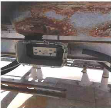
5 1 - Closet/Utility/Mechanical Outlets/Switches - Roof top GFCI non op, missing cover
