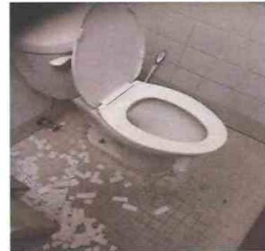
23 1 - Office Floor - Hard - Toilet loose at base in the shop
