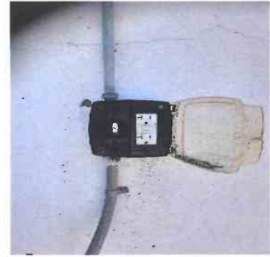
10 1 - Closet/Utility/Mechanical Outlets/Switches - GFCI non op on roof top
