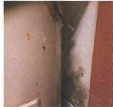
33 1 Unit 1-301 - Local Systems Water Heater - Missing pressure release tube
