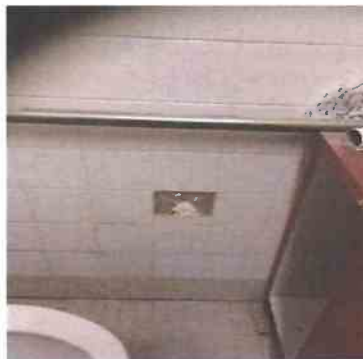
25 1 - Office Walls - Missing tile in the shop bathroom
