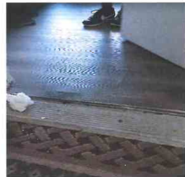
24 1 Unit 1-110 - Living Room Floor - Hard - Tripping hazard entry door
