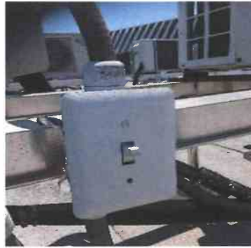
9 1 - Closet/Utility/Mechanical Outlets/Switches - Switch missing cover on roof top
