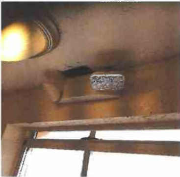
1 - Halls/Corridors/Stairs Lighting - Missing cover on aux lighting, second floor staircase.
