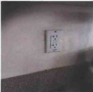
14 1 Unit 1-102 - Kitchen Outlets/Switches - Loose GFCI.
