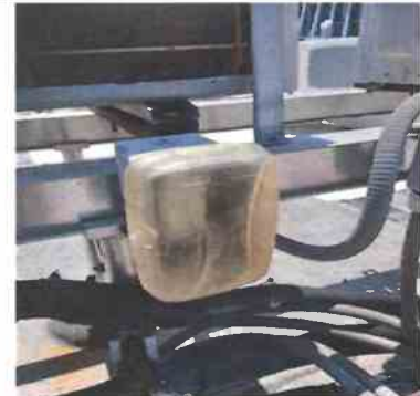
7 1 - Closet/Utility/Mechanical Outlets/Switches - GFCI non op on roof top
