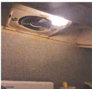
25 1 Unit 1-205 - Kitchen Range Hood/Vent Fan - Missing vent fan cover
