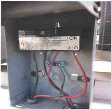
3 1 - Electrical Electric Panel - Missing plate for 103 on roof top
