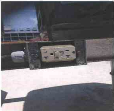
6 1 - Closet/Utility/Mechanical Outlets/Switches - Roof top GFCI missing plate/cover, GFCI non op
