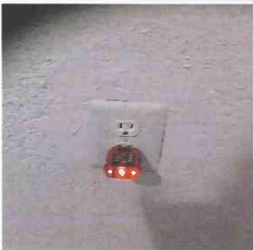
16 1 Unit 1-101 - Living Room Outlets/Switches - Improper wiring configuration back wall
