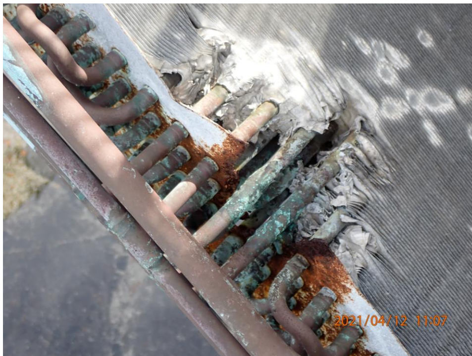
Condenser Coil on RTU
