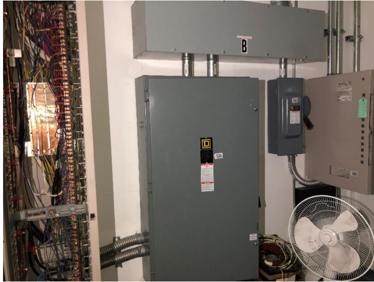
Electrical Disconnect and Wireway for Stage Dimming Equipment
