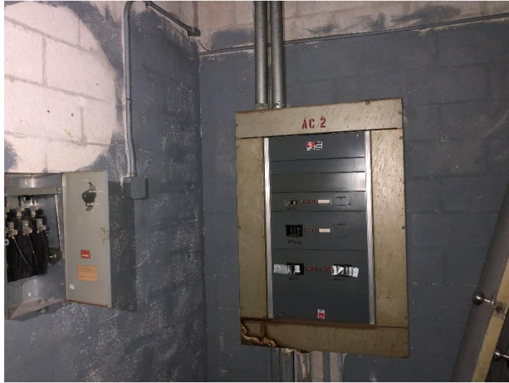
Electrical Distribution Panel for Air Conditioning Equipment
