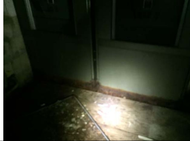
0.5 Flood line on wall in switchgear room
