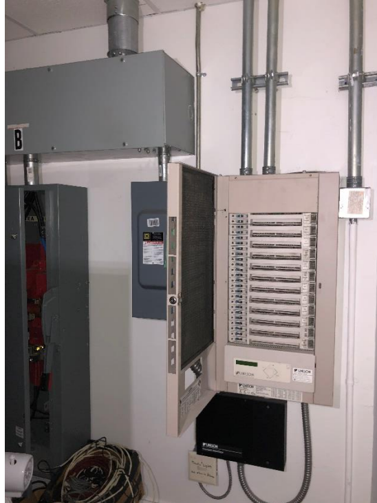
Stage Dimming Equipment
