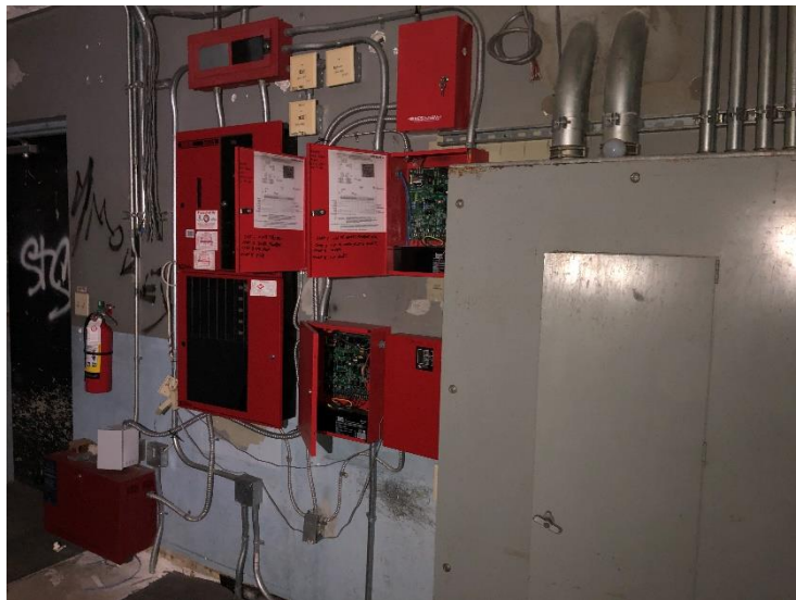
Fire Alarm Equipment
