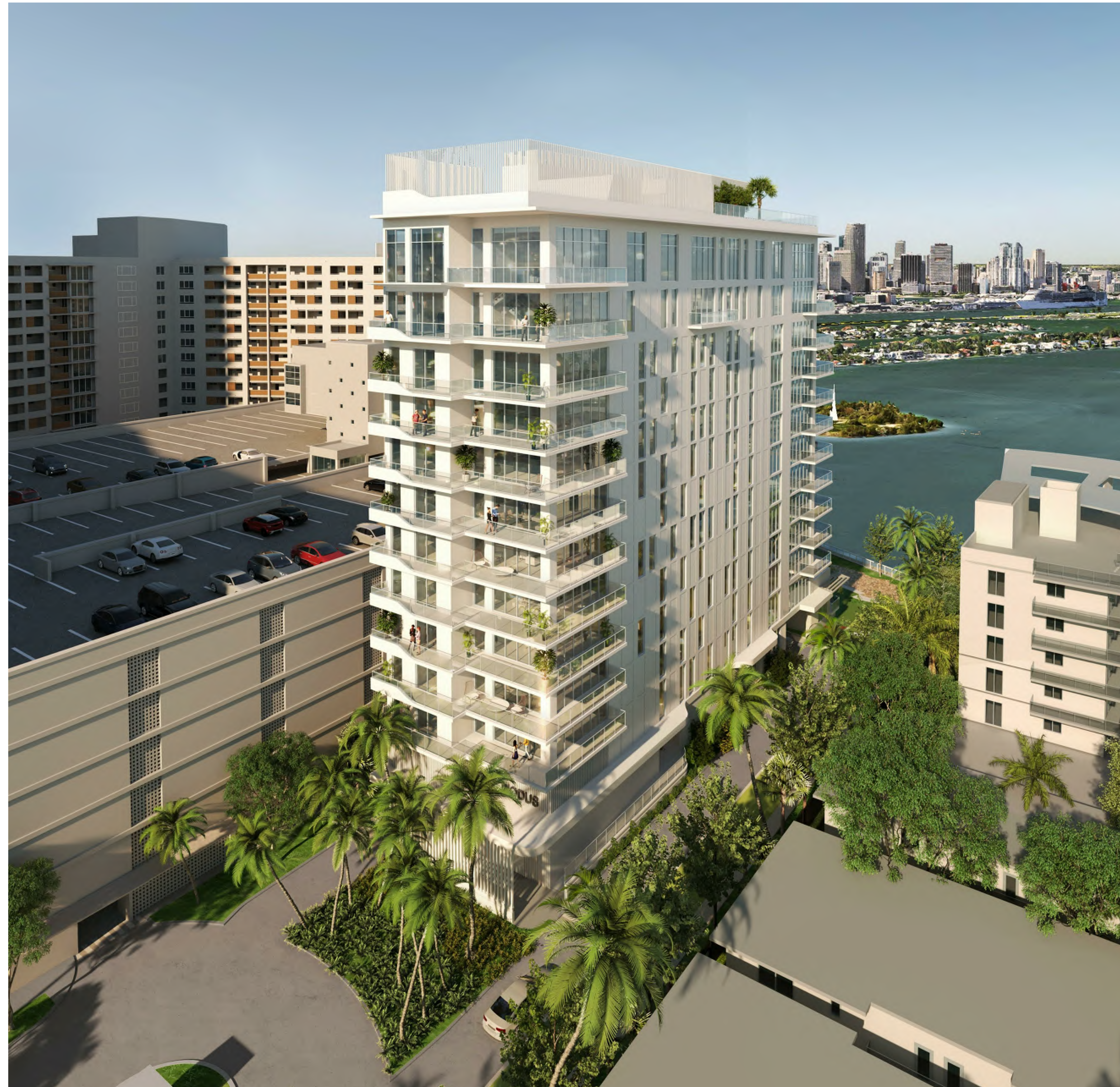
VIEW FROM BAY ROAD - FACING NORTHWEST
