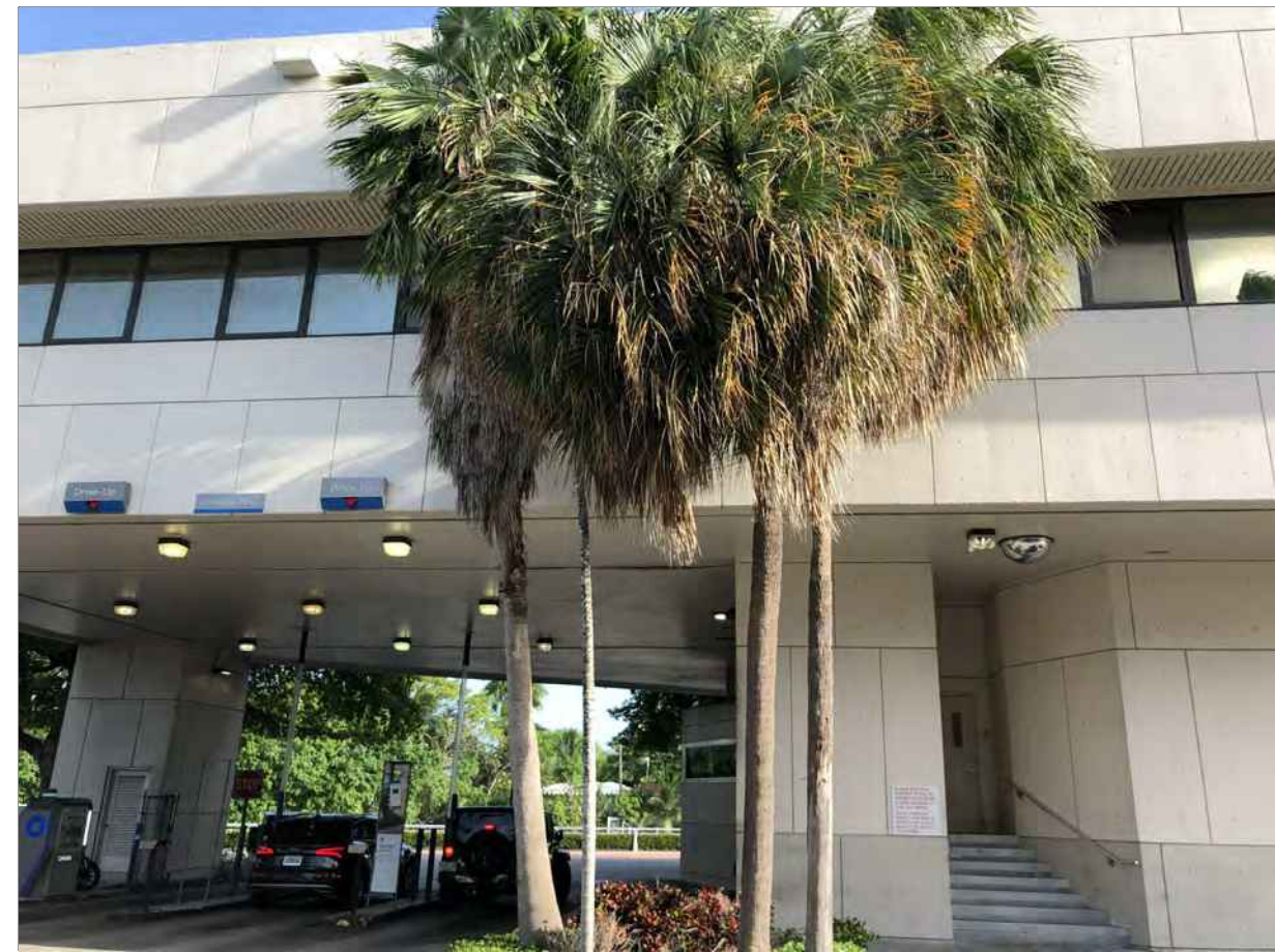
10 EXISTING PARKING LOOKING SOUTH
