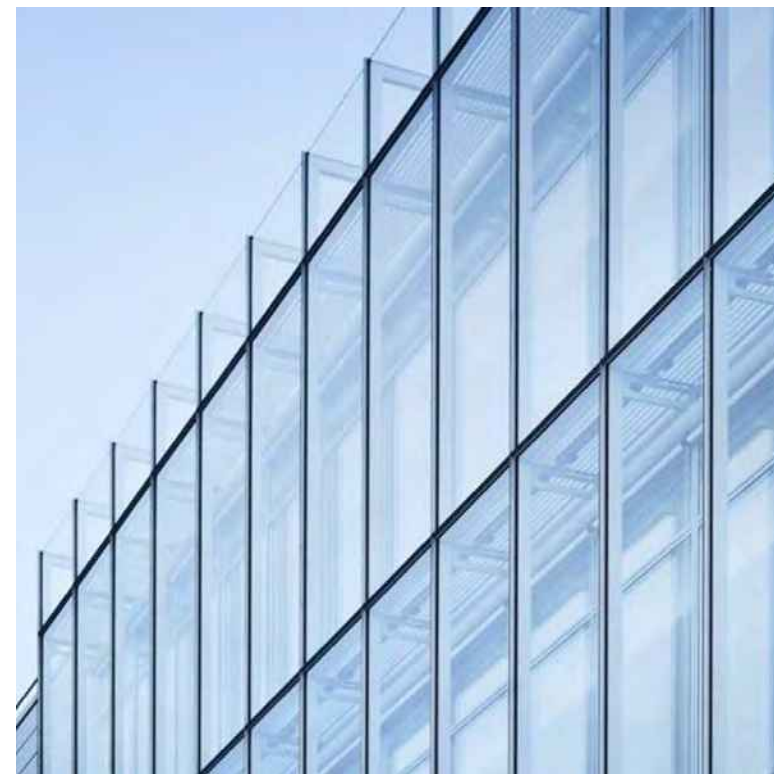
02 LOW E CLEAR INSULATED GLAZING WITH LIGHT U/V TINT
