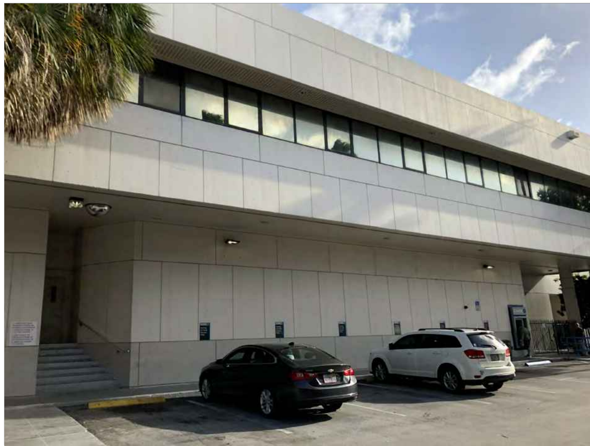
09 EXISTING PARKING LOOKING SOUTHWEST
