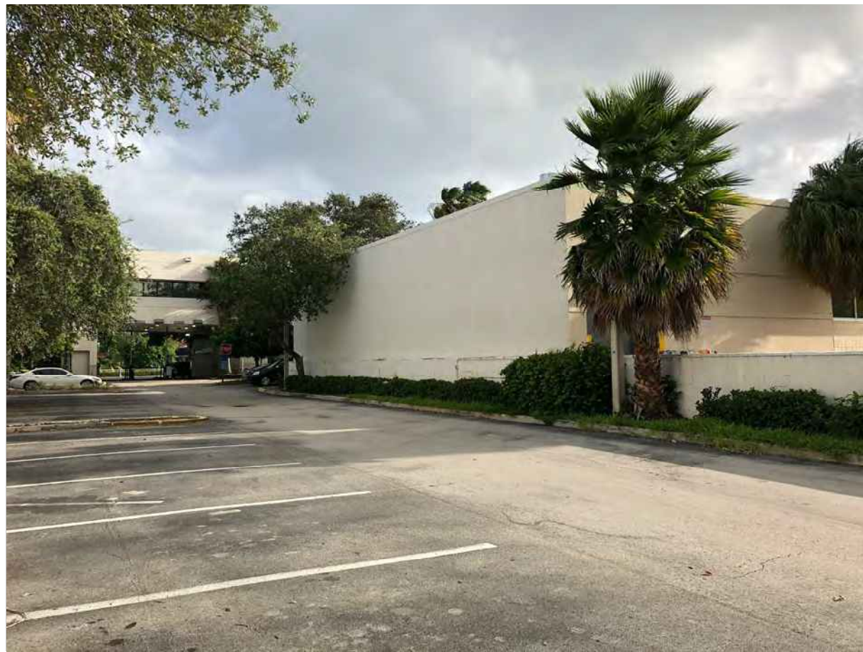
13 EXISTING PARKING LOOKING SW
