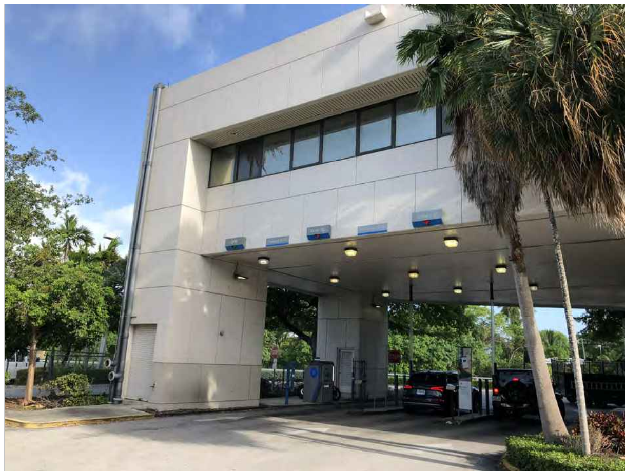
11 EXISTING PARKING LOOKING SOUTHEAST
