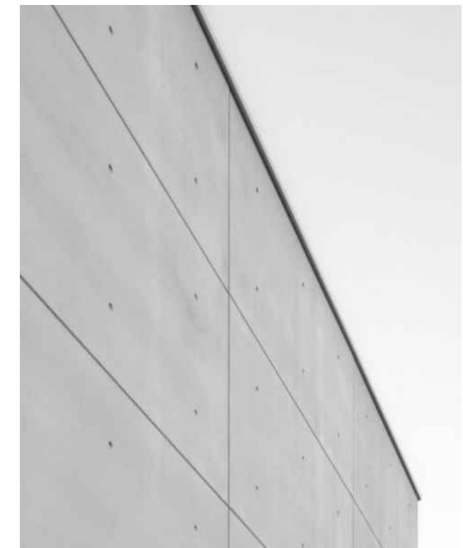
01 CAST IN PLACE ARCHITECTURAL CONCRETE
