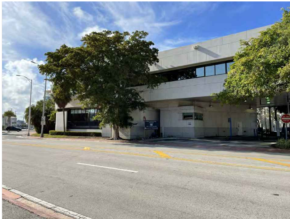
05 DADE BOULEVARD LOOKING NORTHWEST
