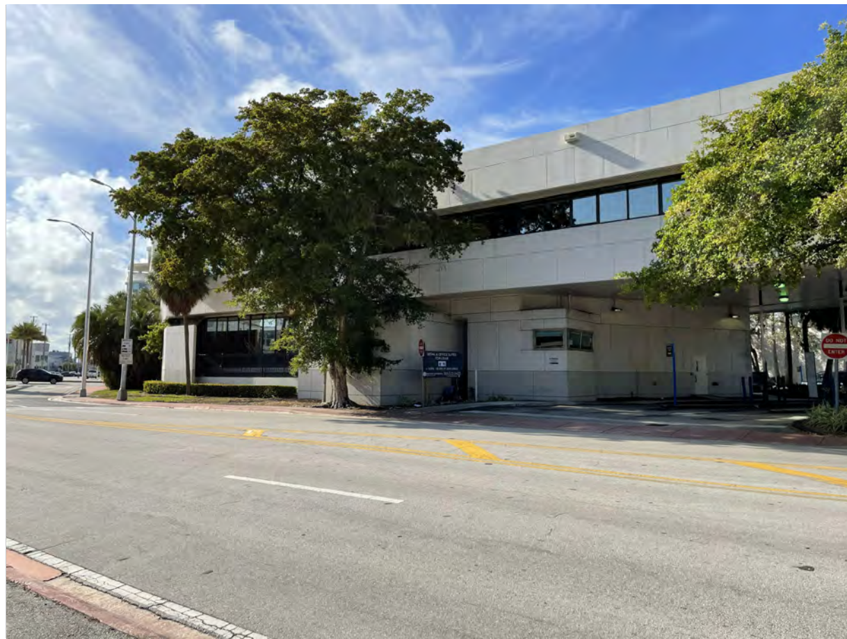
05 DADE BOULEVARD LOOKING NORTHWEST
