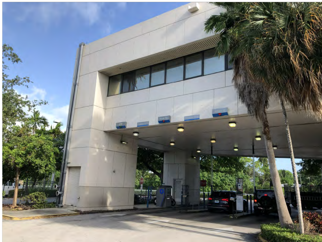
11 EXISTING PARKING LOOKING SOUTHEAST
