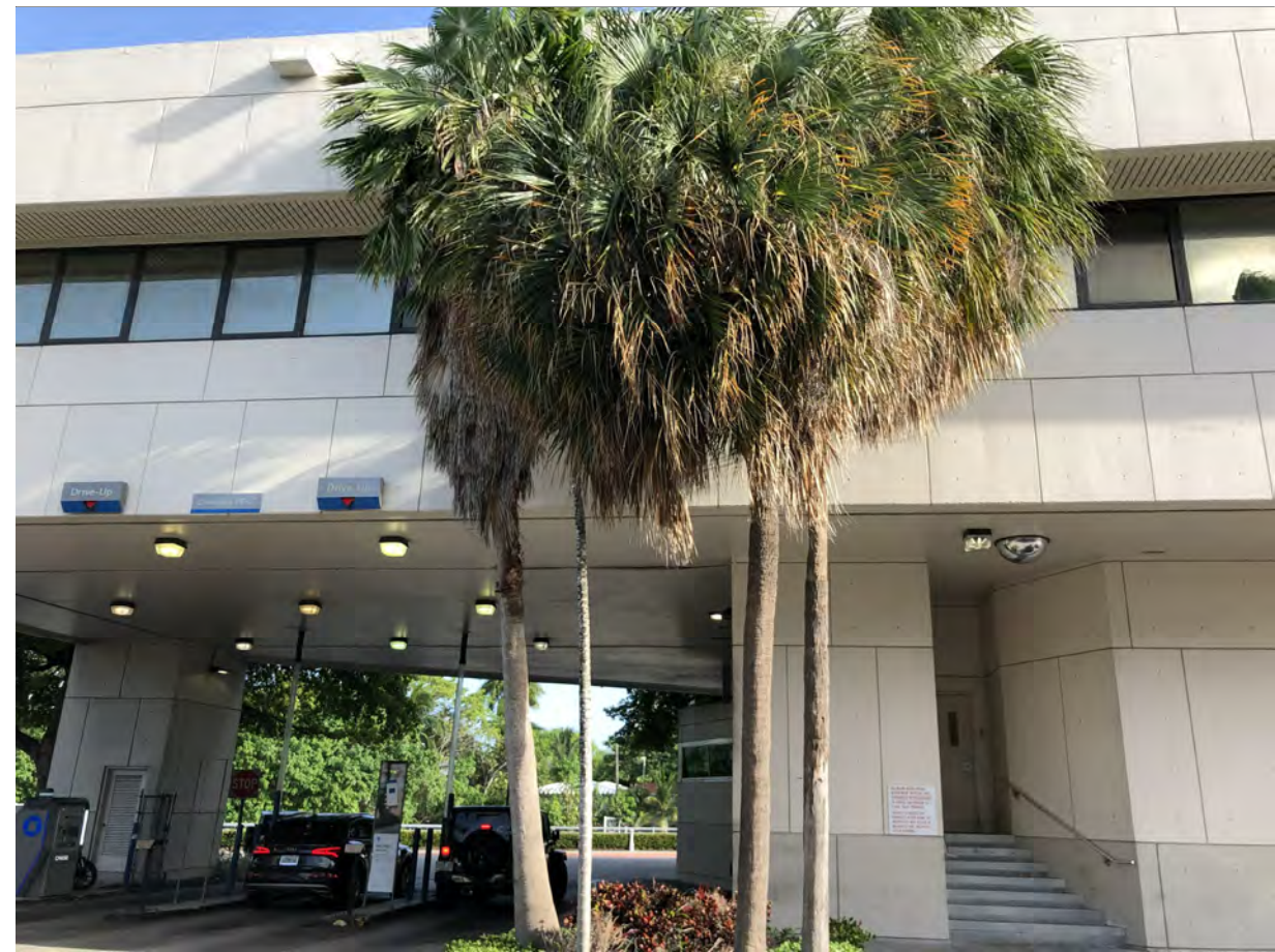
10 EXISTING PARKING LOOKING SOUTH
