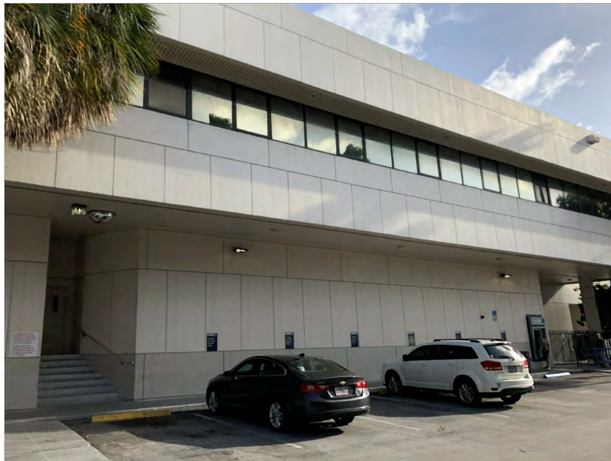
09 EXISTING PARKING LOOKING SW
