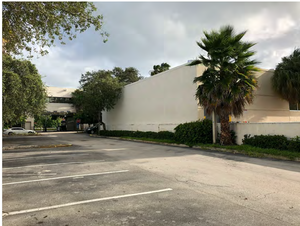
13 EXISTING PARKING LOOKING SW
