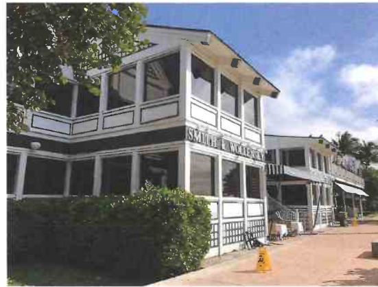
Photo 2 – Rear Elevation from Bay Walk
