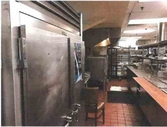
Photo 13 – 2 nd Floor Kitchen
