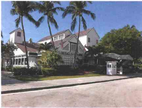
Photo 1 – Front Elevation & Entrance
