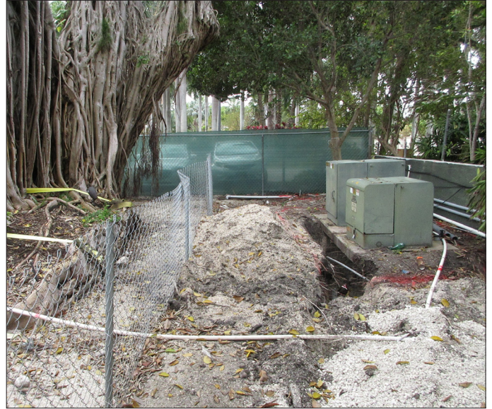
Trenching around electrical boxes
