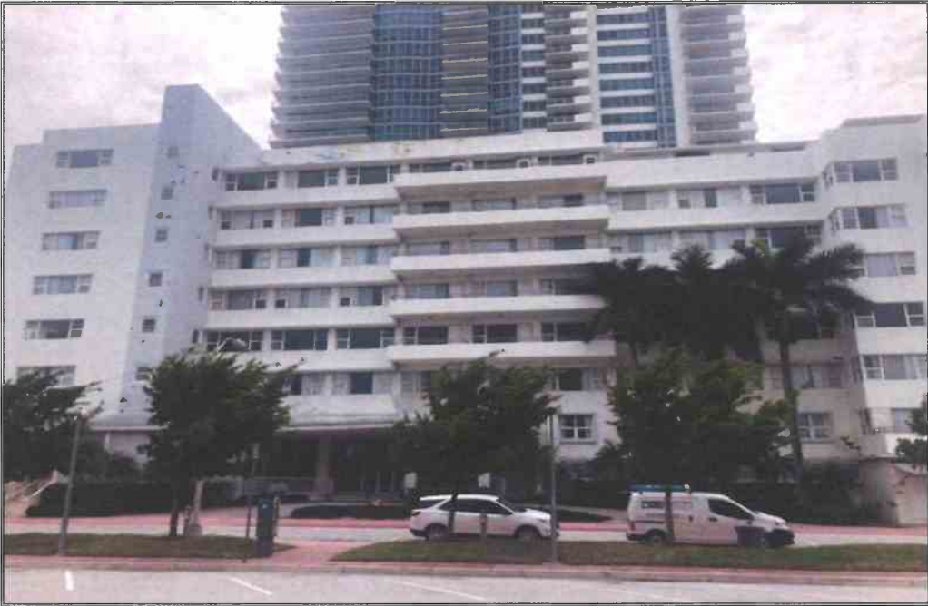
NORTH SIDE OF EXISTING HOTEL FACING SOUTH AT 21 ST STREET
