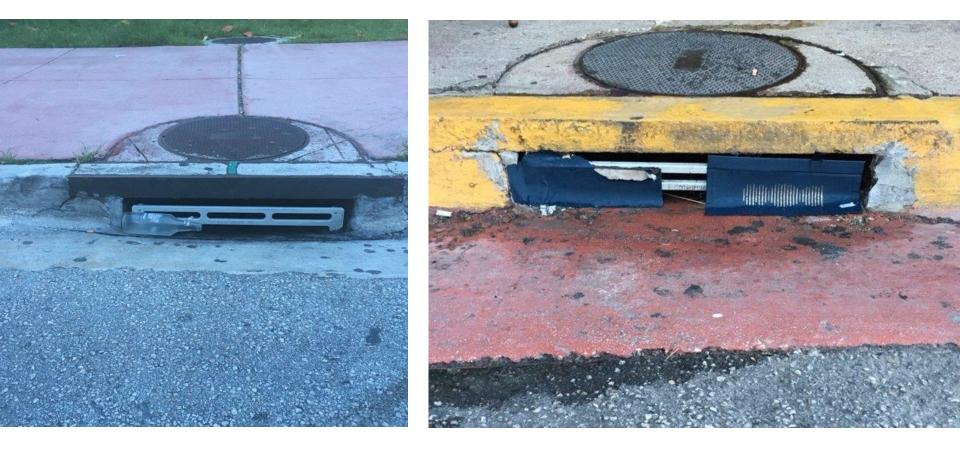
Figure 4: EcoSense grates are better for stopping larger items but need to be cleaned frequently by street sweepers.
