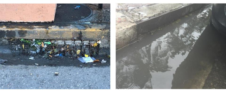
Figure 2: Stop Ocean Pollution Grates clogged with trash and debris do not look aesthetically pleasing in between cleanings.
