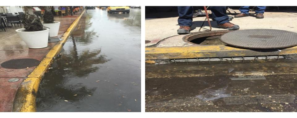
Figure 3: Grates clog and backup water into the street.
