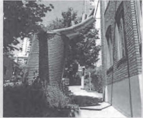
The ten-foot-high Beckoning Cistem distributes water down the hill in a series of cascading planters when it becomes full.
