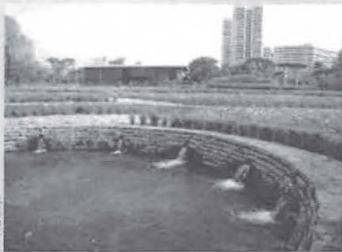
The cleansing biotopa helps filter the water before it is returned to the drainage system in the park.
