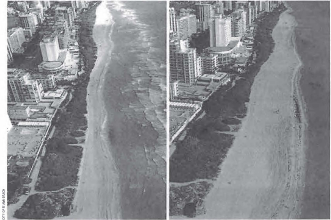
Miami-Dade County Beach Erosion Control and Hurricane Surge Protection Project deposited 18,500 truck-hauls of sand in Miami Beach in 2016 alone. Depicted are the beach before (left) and after the protection project.
