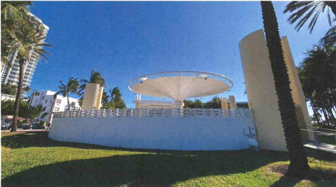
Current photograph of the bandshell complex showing recently installed canopy
