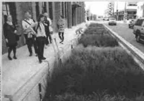
A rain garden acts as a sponge, helping water permeate the ground naturally while also nurturing the landscaped plants.
