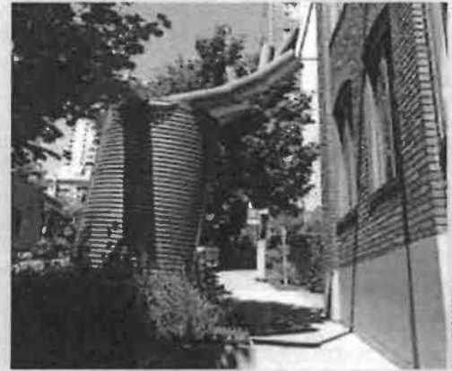
The ten-foot-high Beckoning Cistem distributes water down the hill in a series of cascading planters when it becomes full.
