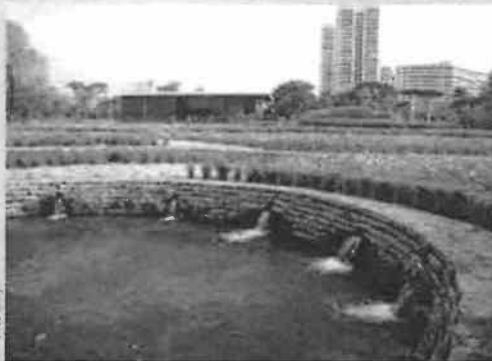
The cleansing biotope helps filter the water before it is returned to the drainage system in the park.
