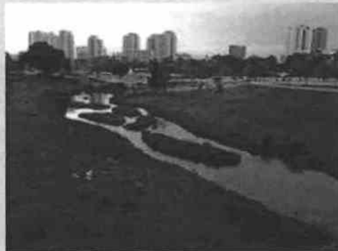
The Kallang River was removed from its concrete encasing and now can widen up to 330 feet in flood conditions, increasing conveyance by 40 percent.
