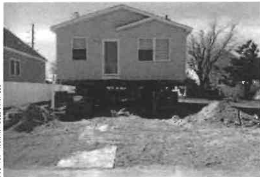
A community adaptation fund would assist residents with making the necessary improvements to their homes to protect them, as with this elevated home in the Northeast.
