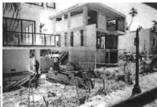
New construction in Miami Beach is designed with living space well above ground, allowing the ground floor to flood.
