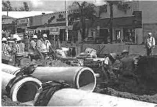
The current program has installed new drainage pipes throughout the city, such as this one on Alton Road.
