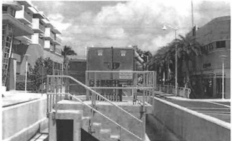
Newly installed stormwater infrastructure can be seen here in Sunset Harbour.
