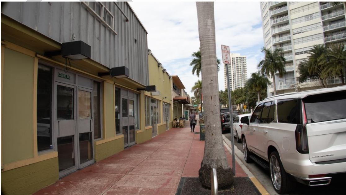
Figure 29: Existing condition of a streetscape
