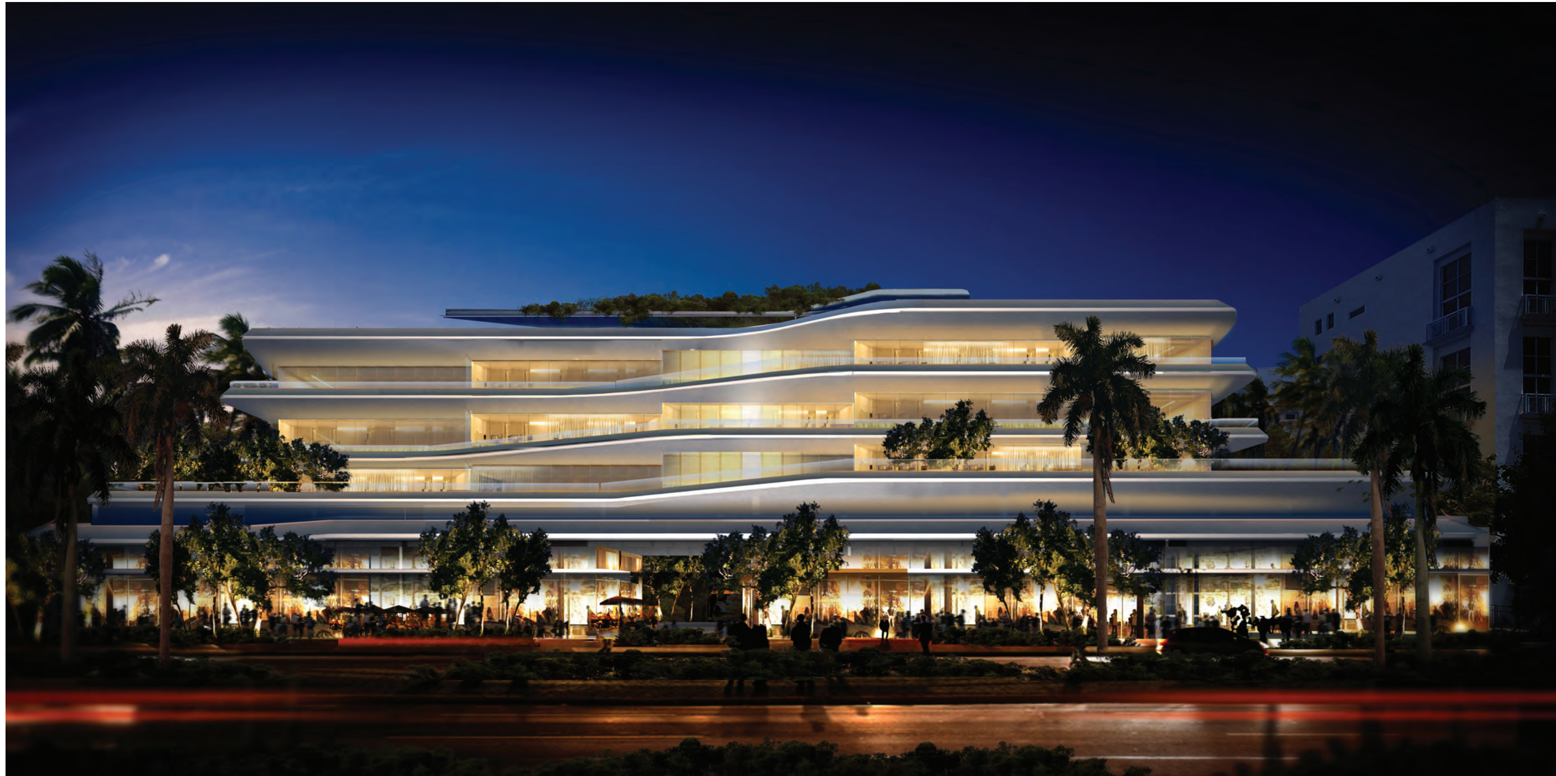
MAIN ENTRY VIEW
