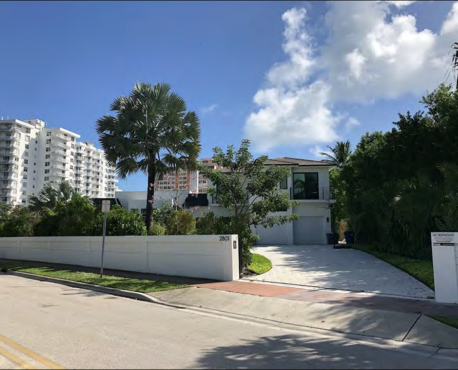
01 2801 FLAMINGO DRIVE (LOOKING EAST)
