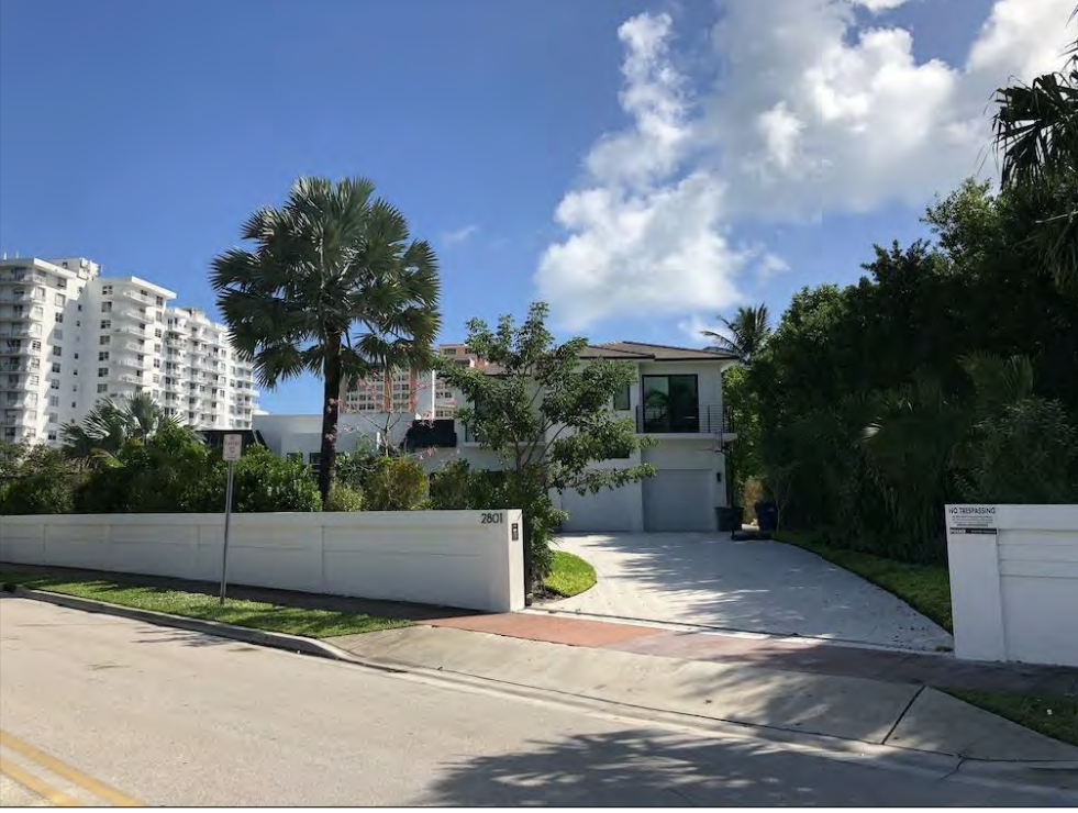
01 2801 FLAMINGO DRIVE (LOOKING EAST)
