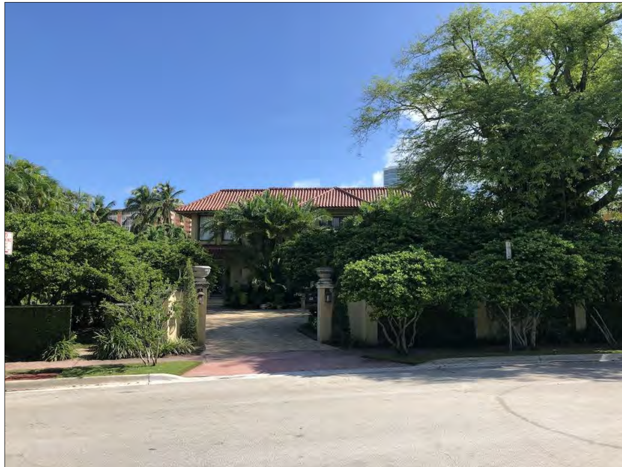
01 2653 FLAMINGO DRIVE (LOOKING EAST)
