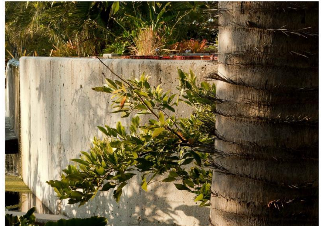
Exposed Concrete Walls
