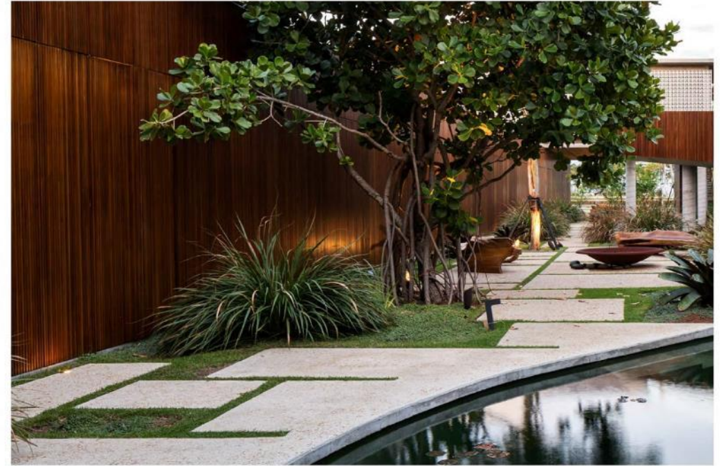
Concrete Stepping Pads with Exposed Aggregate
