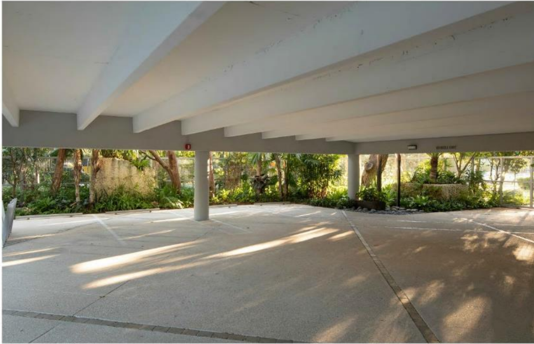
Concrete Driveway with Exposed Aggregate
