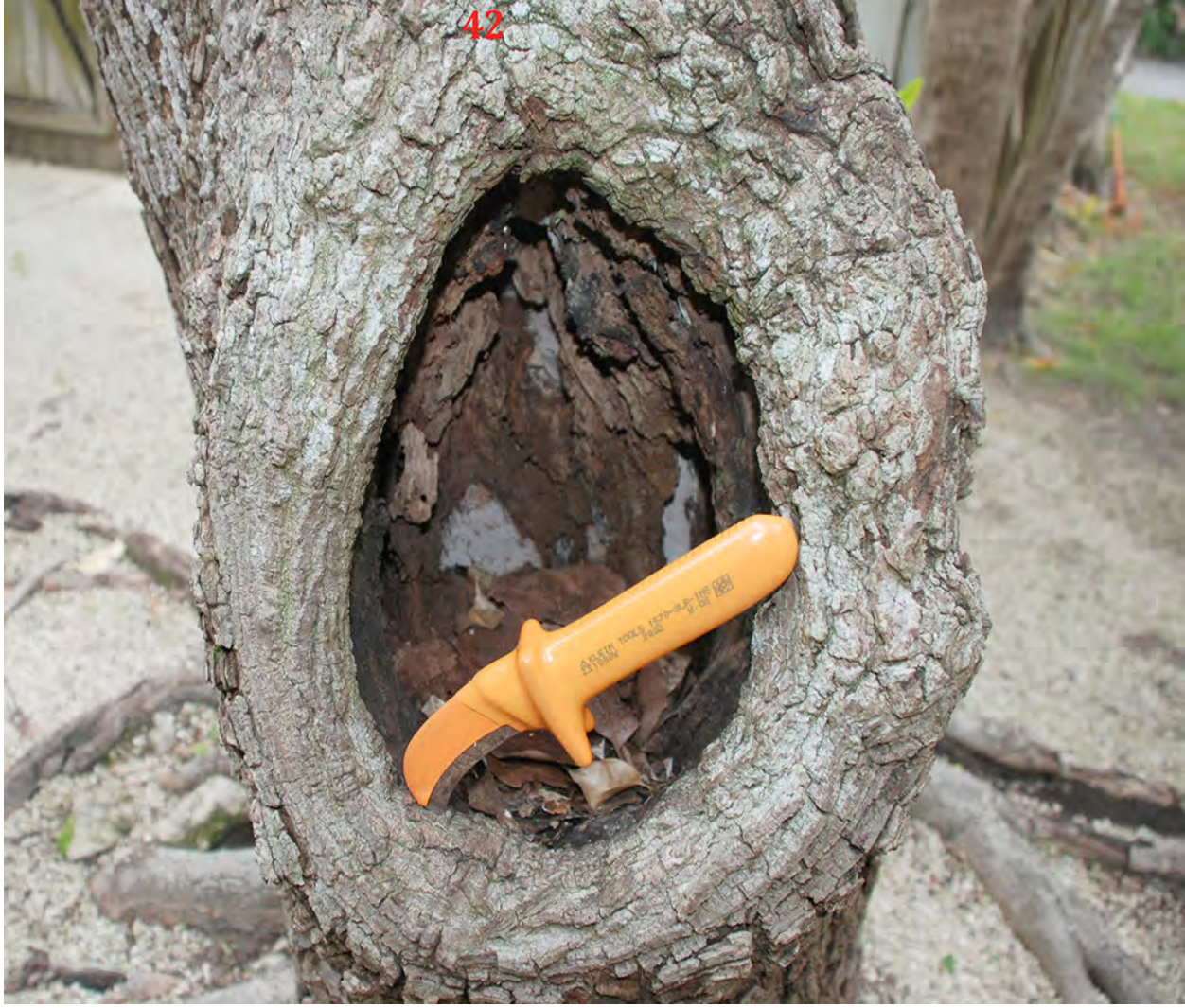
Photo 23 above is a closer view of the large cavity on tree 42. The orange knife is 7 inches in length. This tree should be considered for removal.
