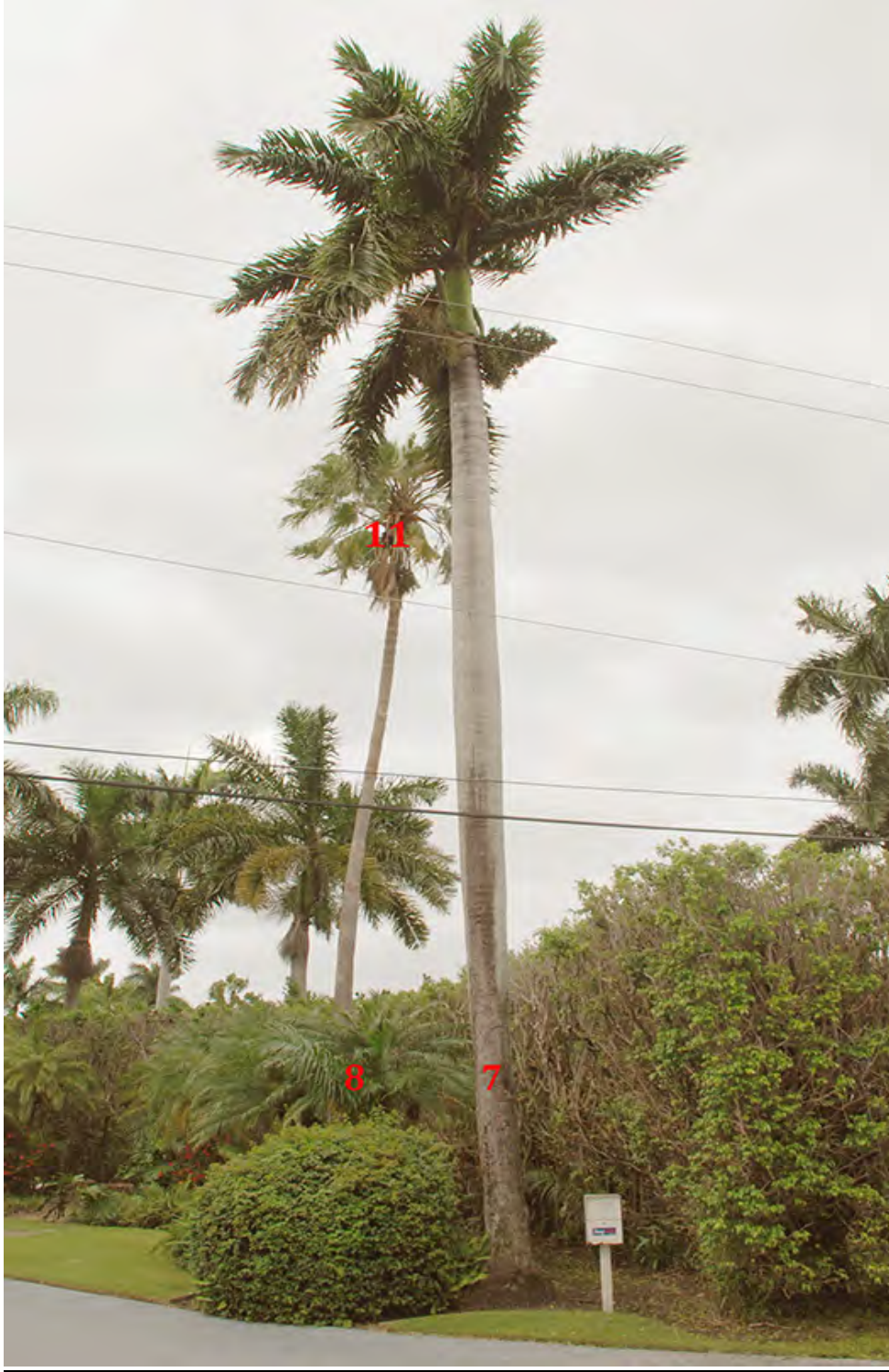
Photo 5 above is palms 7, 8 & 11. Note the adjacent powerlines.
