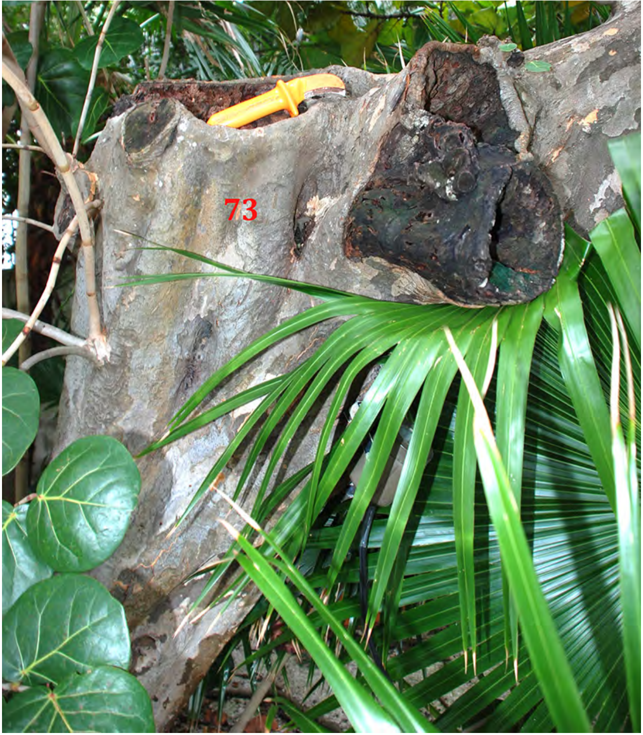
Photo 38 above are two large sections of decay on the north side of the trunk of tree 73 caused by large pruning wounds. This tree should not be considered for relocation.
