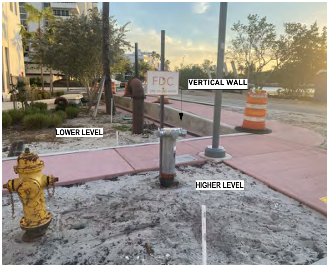
INDIAN CREEK & 33 STREET
