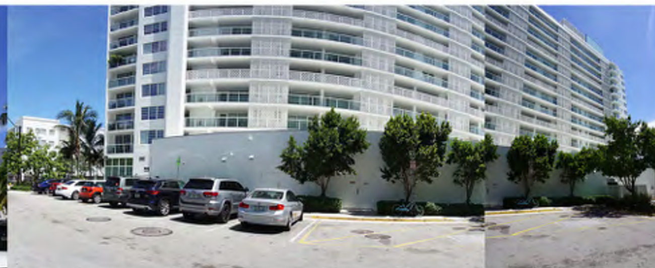
8. NORTH FACADE ALONG 10TH ST. PHOTOGRAPHS TAKEN ON JULY 8TH, 2020
