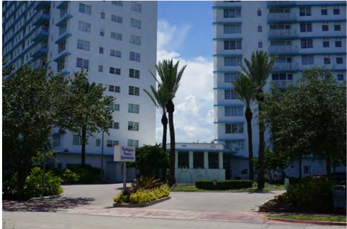
1. ENTRY SIGN. PHOTOGRAPHS TAKEN ON JULY 8TH, 2020
