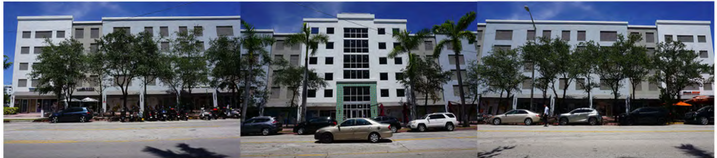
2. RETAIL ACROSS WEST AVENUE. PHOTOGRAPH TAKEN ON JULY 8TH, 2020
