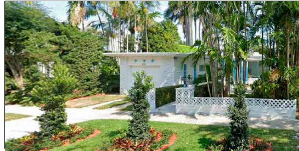
4. 6391 NORTH BAY ROAD
