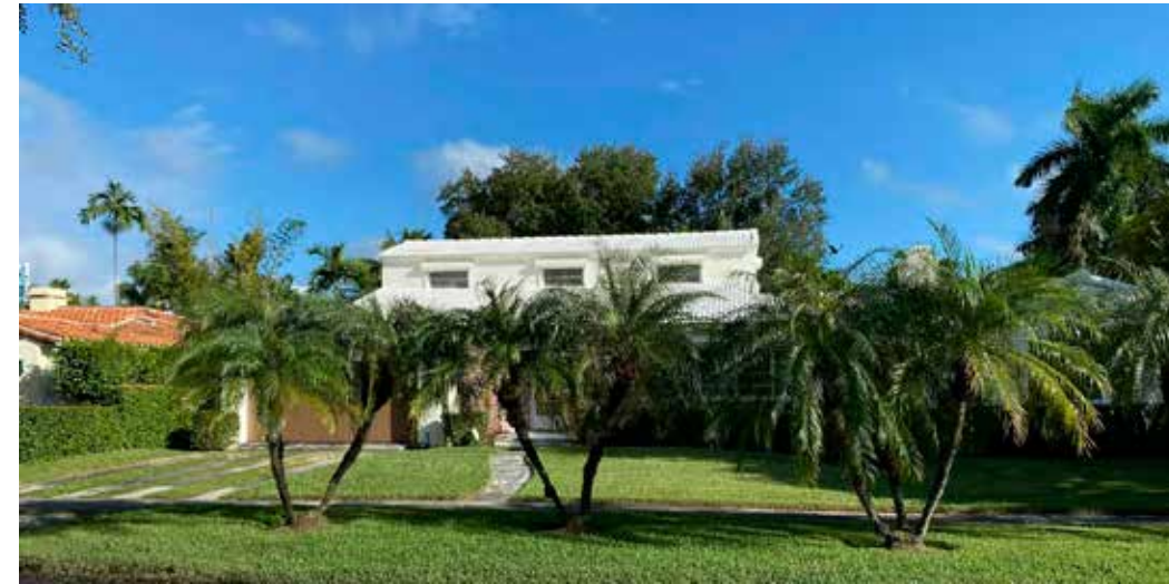
2. 6371 NORTH BAY ROAD
