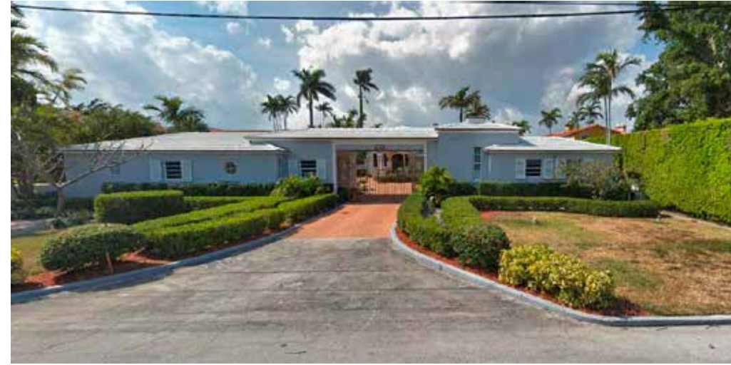
2. 6324 NORTH BAY ROAD
