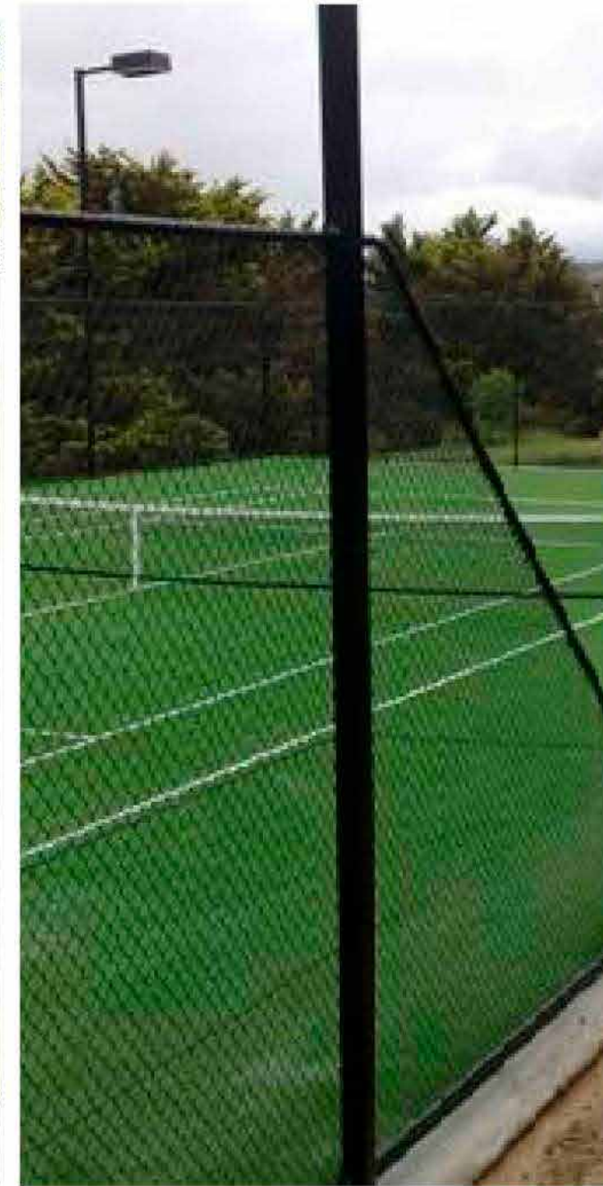
TENNIS COURT FENCE
