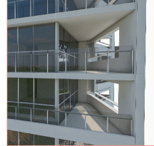
ANODIZED ALUM & GLASS WINDOW-WALL AND BALCONY RAILS
