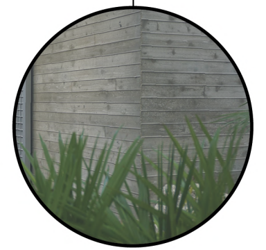
BOARDFORMED CONCRETE
