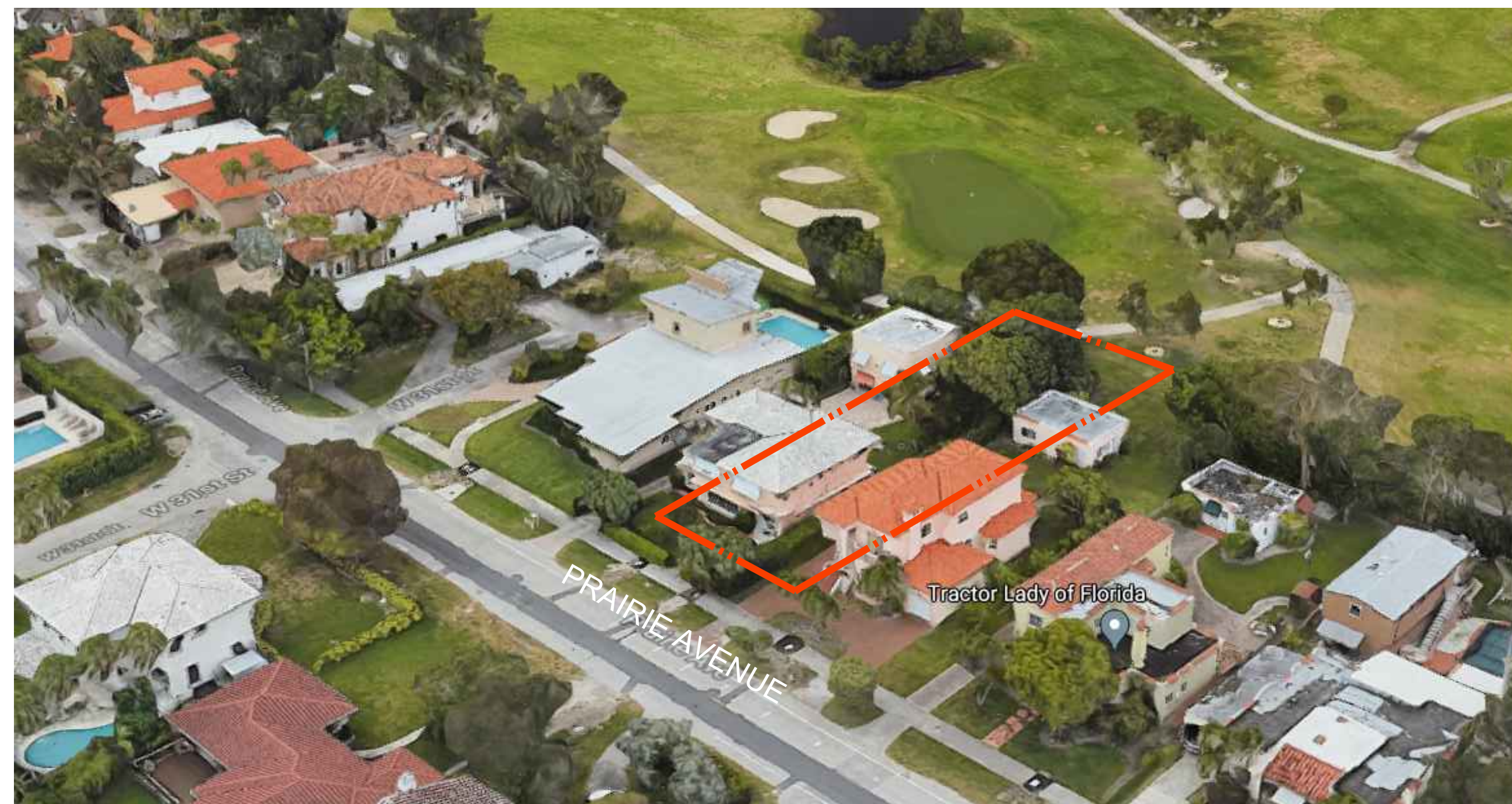
FRONT AERIAL (NE) VIEW
