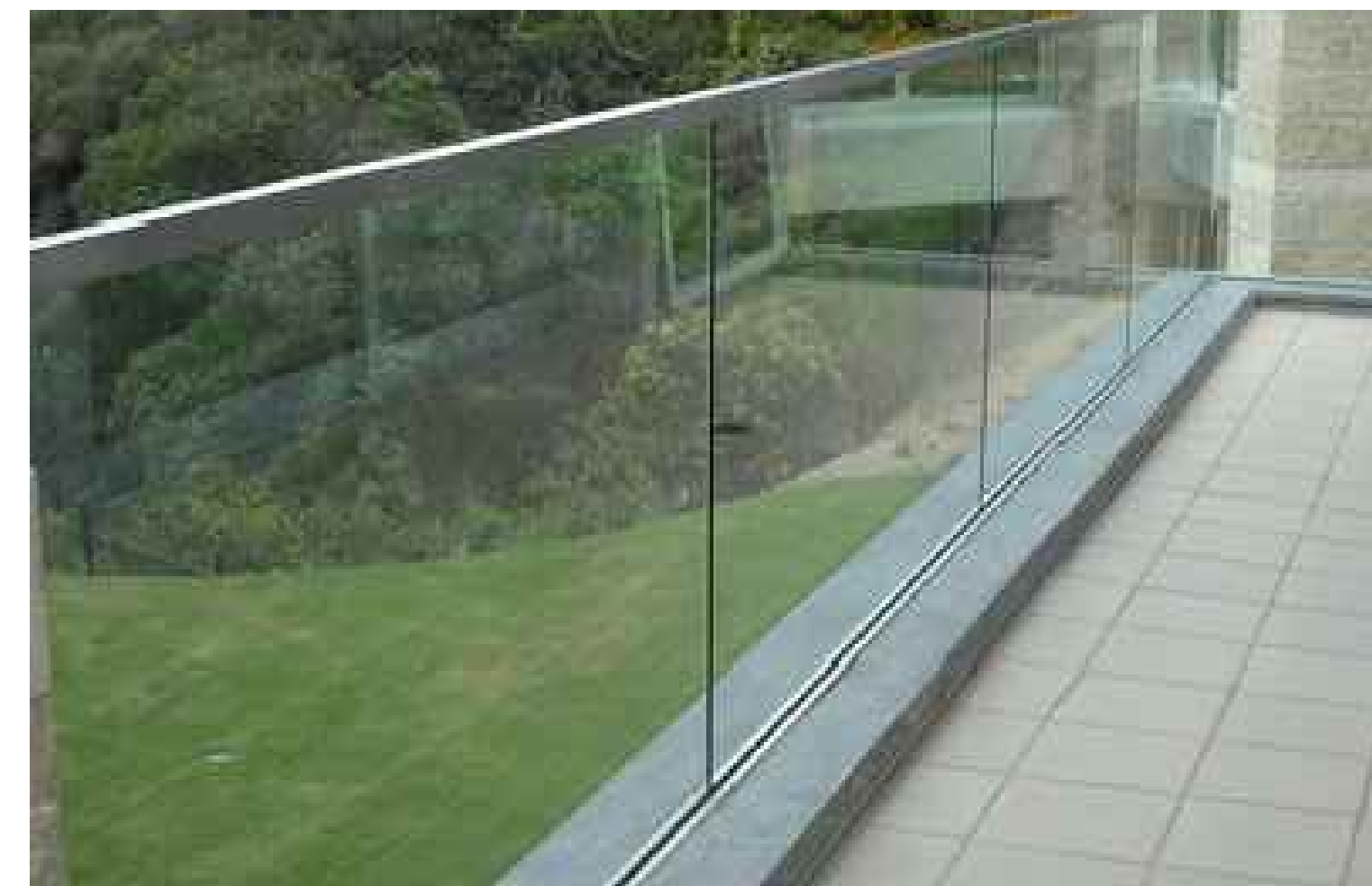
4. LAMINATED GLASS RAILING 42" A.F.F.
