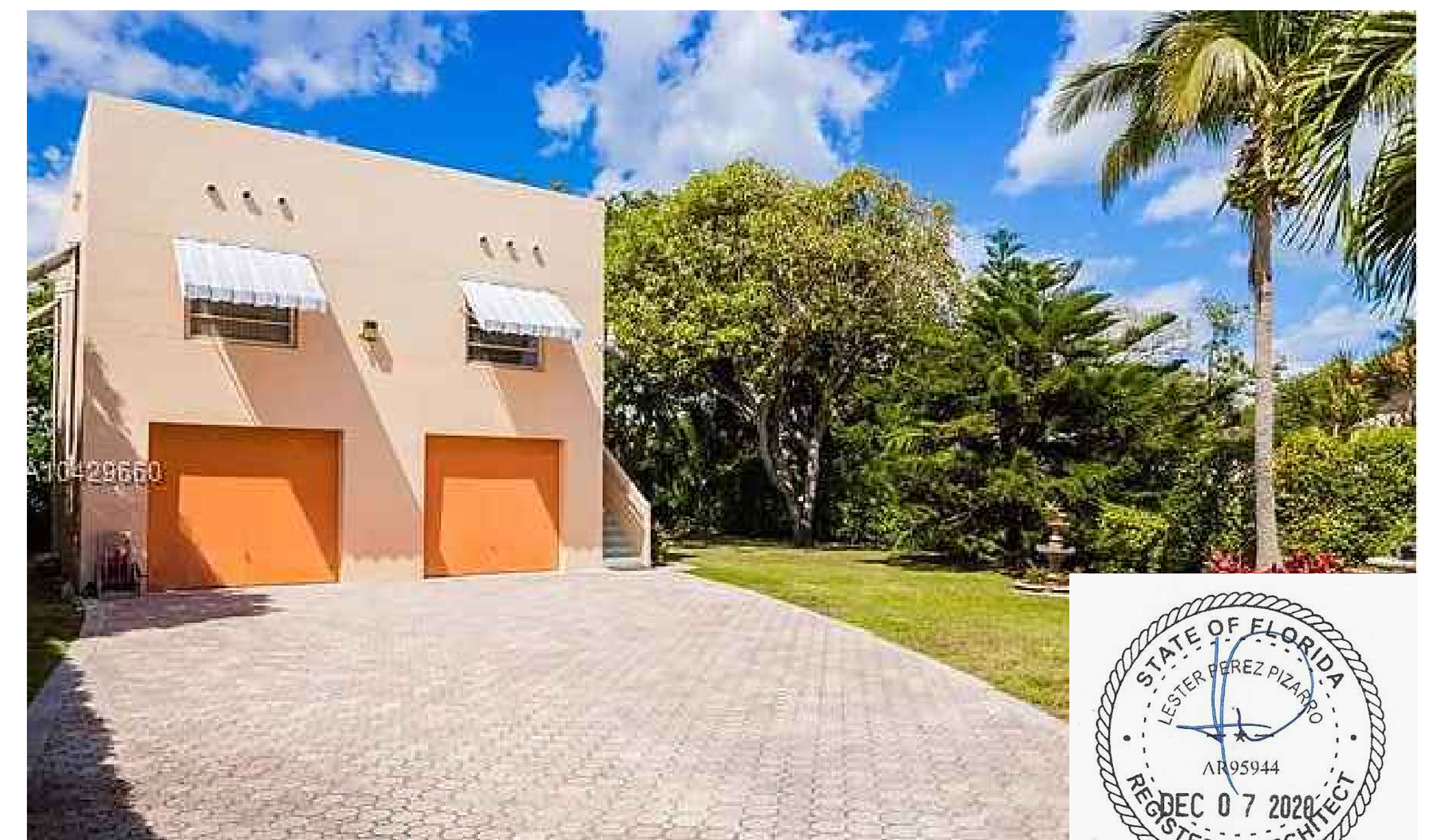
06 REAR ACCESSORY BUILDING VIEW
