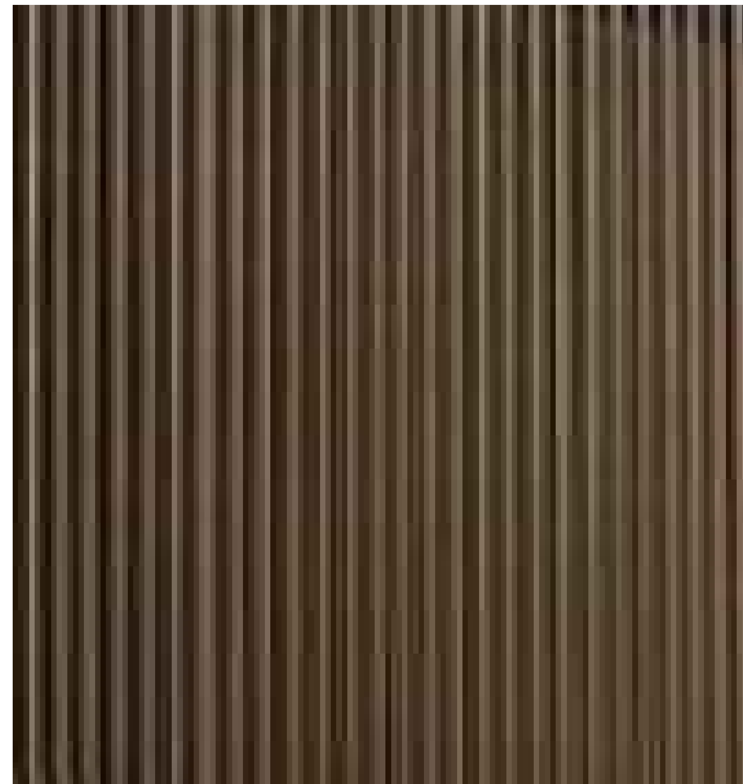
2. ALUMINUM FINNS ON SMOOTH STUCCO WALL PAINTED BRONZE
