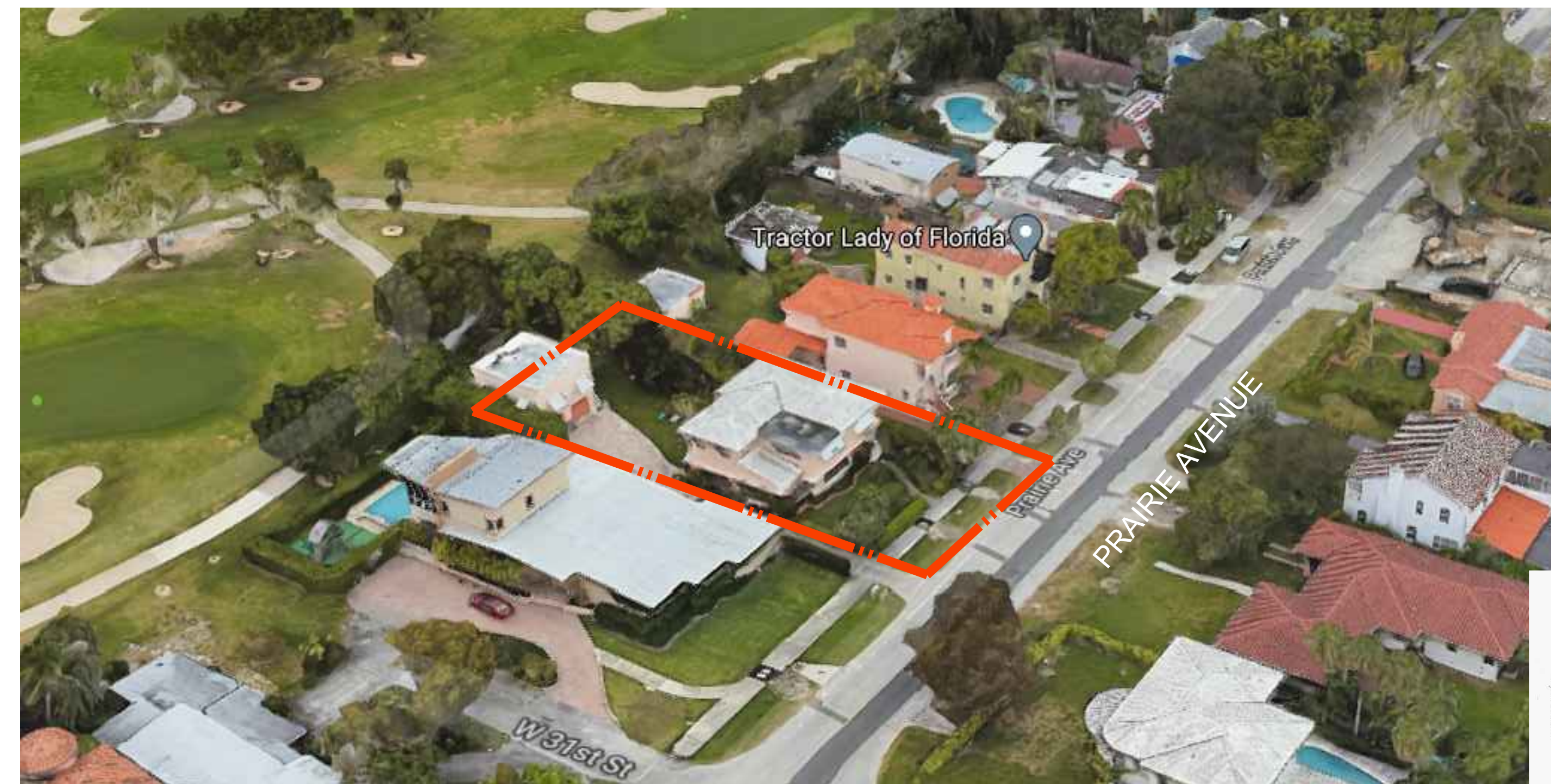
REAR AERIAL (SE) VIEW
